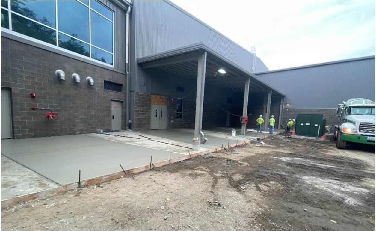
Sidewalks being poured in the kitchen service yard area
