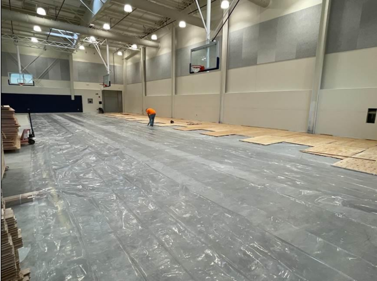
Flooring installation in the Auxiliary Gym
