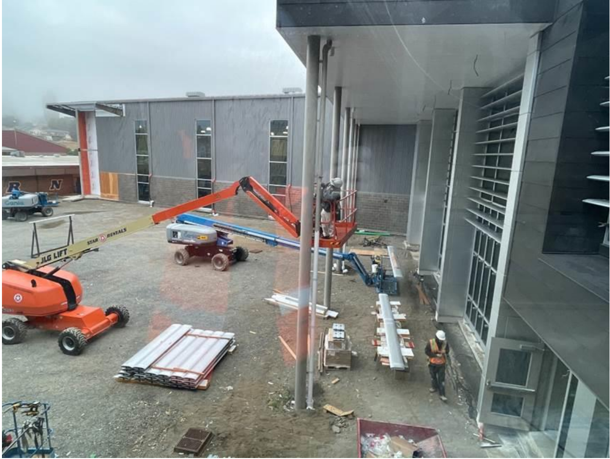
Sun shade installation in the commons area
