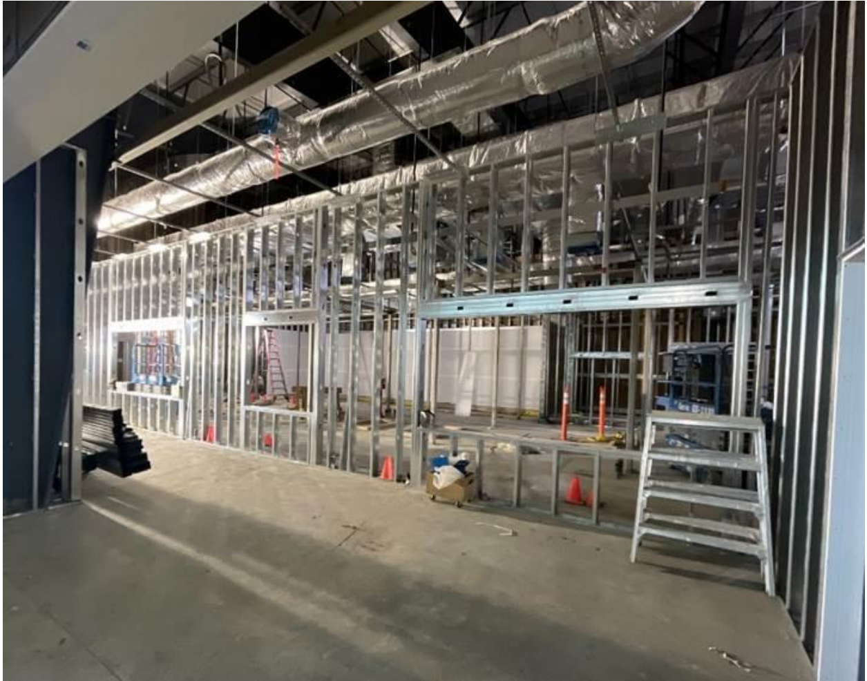
Framed walls at the serving area of the new kitchen
