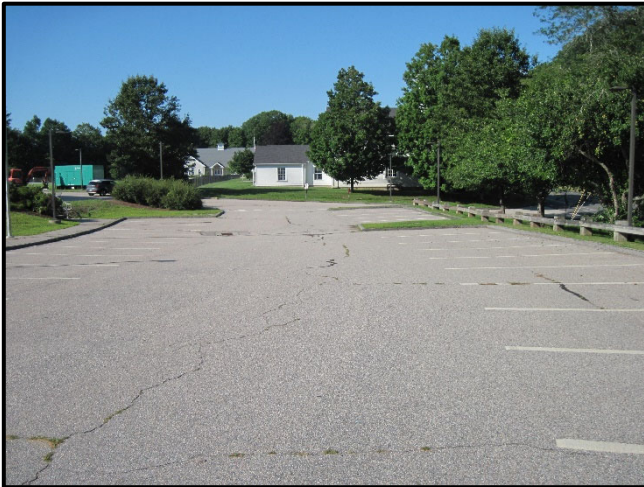
Lot 1 looking north. Various cracks visible in pavement.
