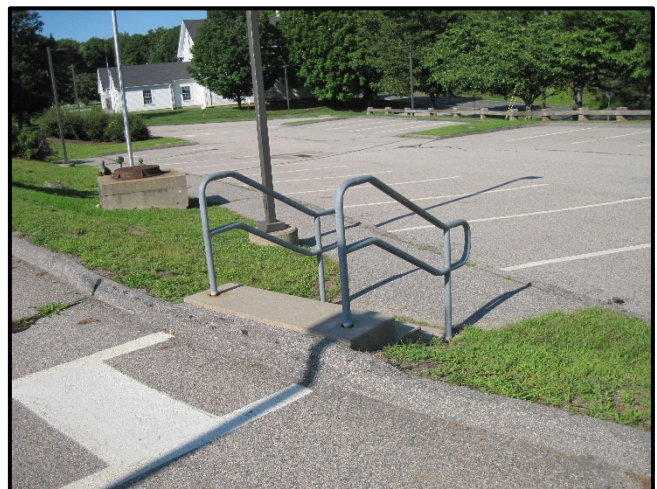
Site stairway "Stair 2" looking northeast. Stairway lacks a landing complying with 2015 IBC 1011.6.
