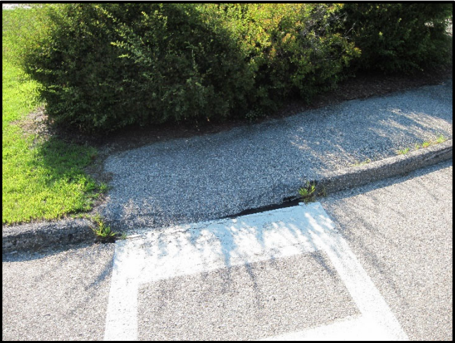
Curb ramp at crosswalk, north end of Lot 1. Ramp is not in compliance with ICC A117.1, 406 (opposing ramp same).
