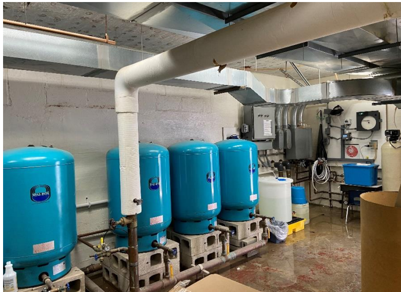
Well Water Storage Tanks
