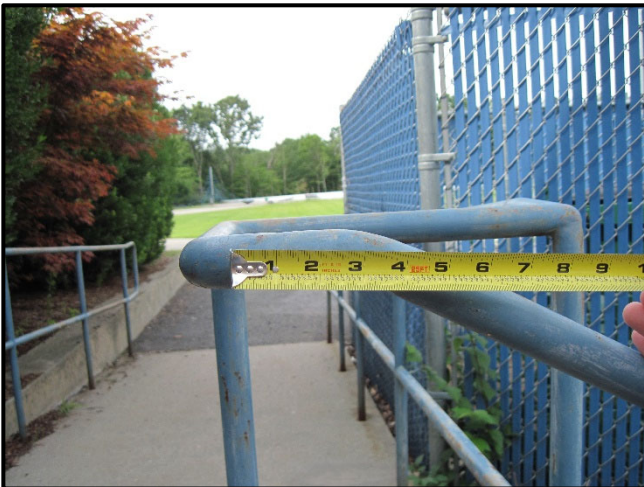
Stair 3, top handrail extension (north rail).
