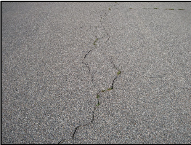
Block cracking with additional cracks propagating.
