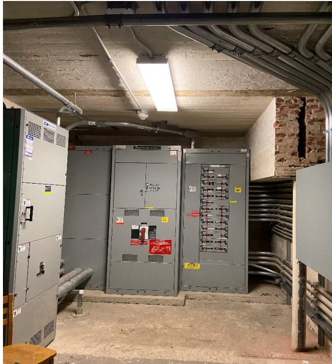
Main Switchboard at Electrical Room
