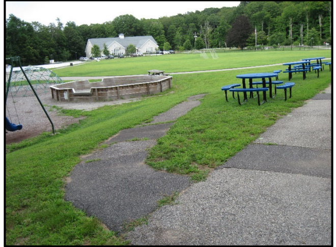
Play Area 2 looking northeast. Bituminous walkway does not comply with ICC A117.1 403.3 (slopes).
