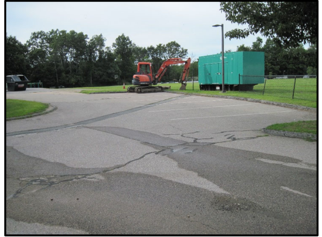
Lot 2 looking north. Generator at edge of Lot 2 visible in background with no vehicle protection.
