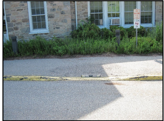
Curb ramp at front of school along bus lane. Ramp is not in compliance with ICC A117.1, 406.
