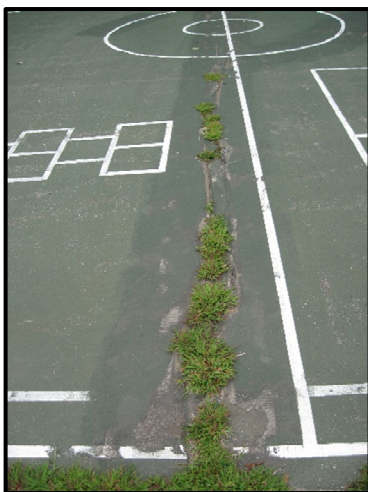
Cracks in basketball court surface. Previous repairs apparent.
