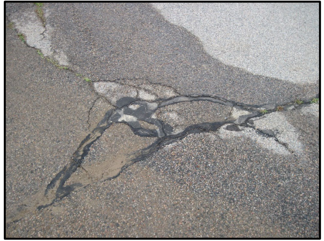
Example of localized fatigue cracking.
