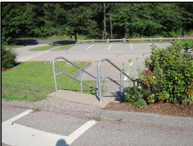
Site stairway "Stair 1" looking east. Stairway lacks a landing complying with 2015 IBC 1011.6.
