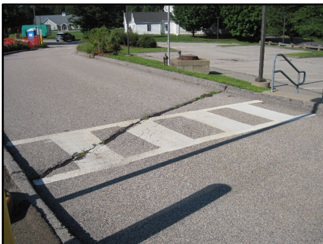
Drive 2 at south pedestrian crossing, large crack visible extending through pavement and bituminous curbs.
