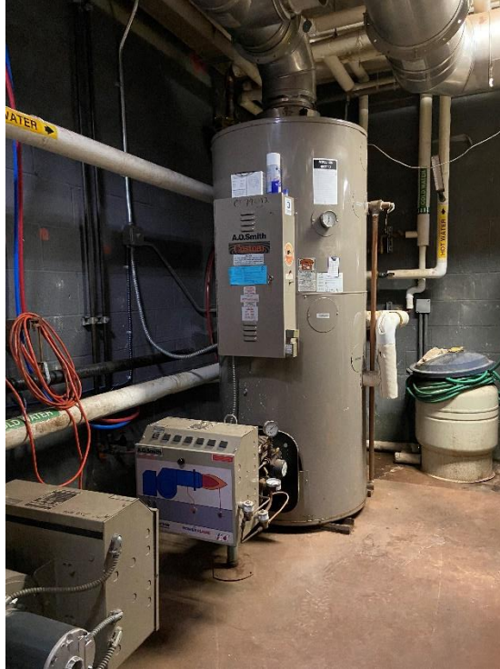
Fuel Fired Water Heaters
