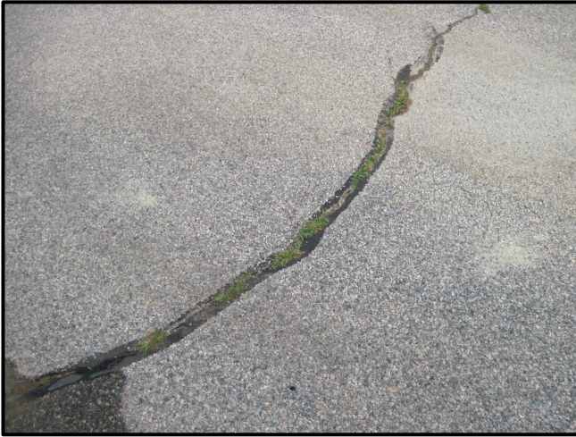
Example of previously repaired crack in bituminous pavement.
