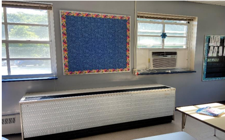
Unit Ventilator Serving a Classroom
