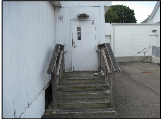
Stairs at Door 11 to portables. Lack of lower handrail extensions and returns visible.
