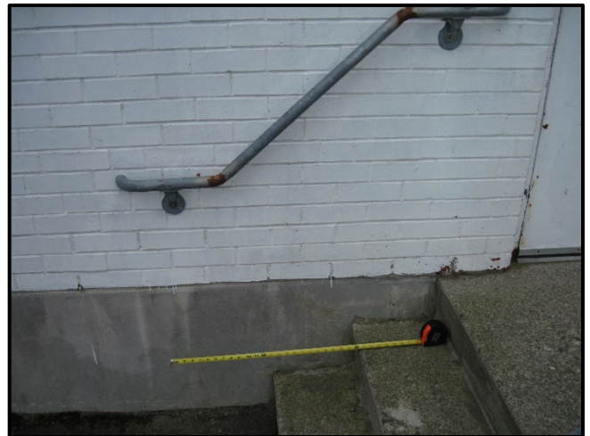
Lower handrail extension at stair railing to Door 10; west rail.
