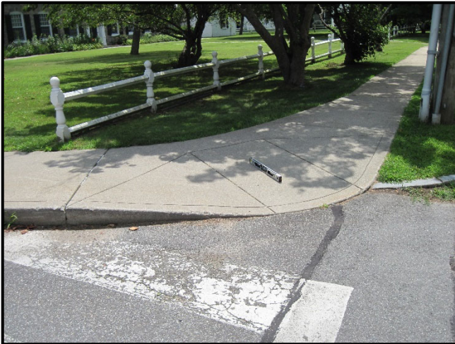
Curb ramp at Lyme Street and Center School Drive 1. Ramp slope >1:12 and does not have a top landing.
