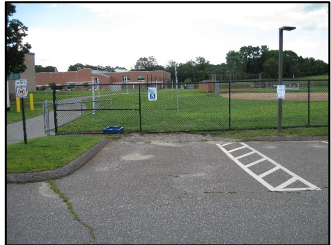
Accessible parking "HC1" at southwest corner of Lot 1. Access aisle not connected to "Accessible Route".
