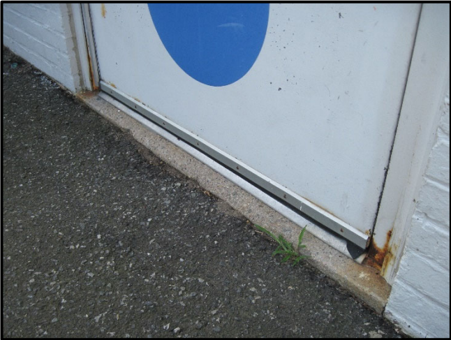
Floor differential at Door 4. Door does not comply with ICC A117.1 404.2.3 for maneuvering clearance.
