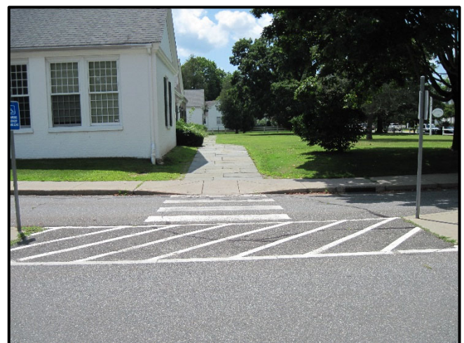
Curb ramp and slate walkway beyond looking west. Ramp slope >1:12 and does not have a top landing.
