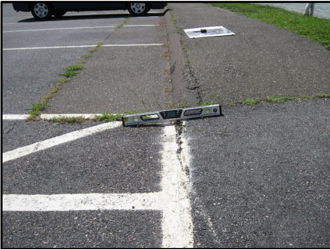
Curb ramp at accessible parking "HC1" connected to bituminous sidewalk along south side of building.
