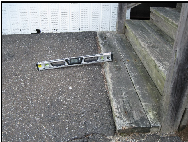
Grade differential at lower landing, stairs at Door 11.
