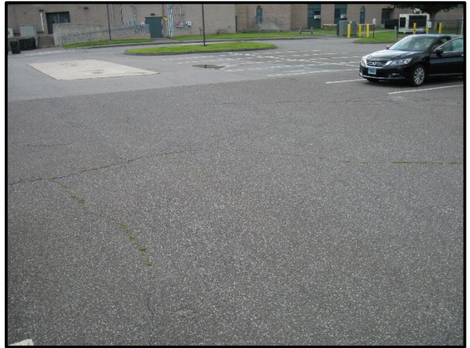
Lot 1 looking east. Fatigue cracking visible. Underground storage tank pad at left/rear of photo.
