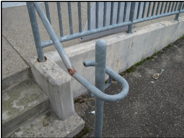
Lower handrail extension and return at stair railing to Door 10; east rail.
