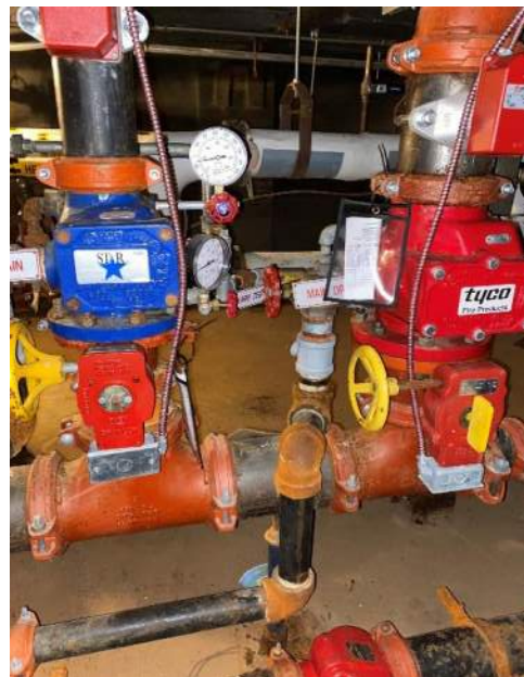
Fire alarm wiring on FP services
