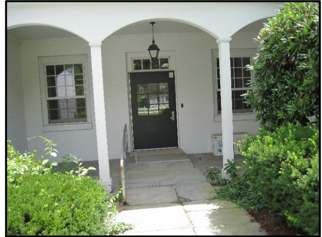
Bluestone ramp at Door 2. Ramp >1:12 . Door does not comply with ICC A117.1 404.2.3.
