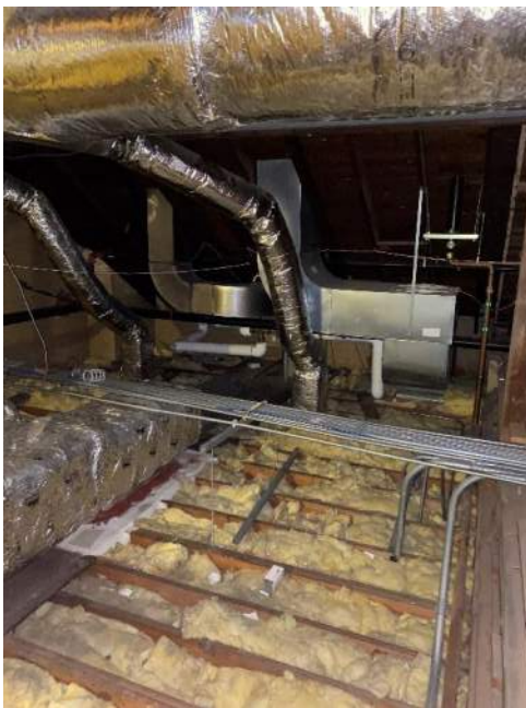
Attic wiring and conduit
