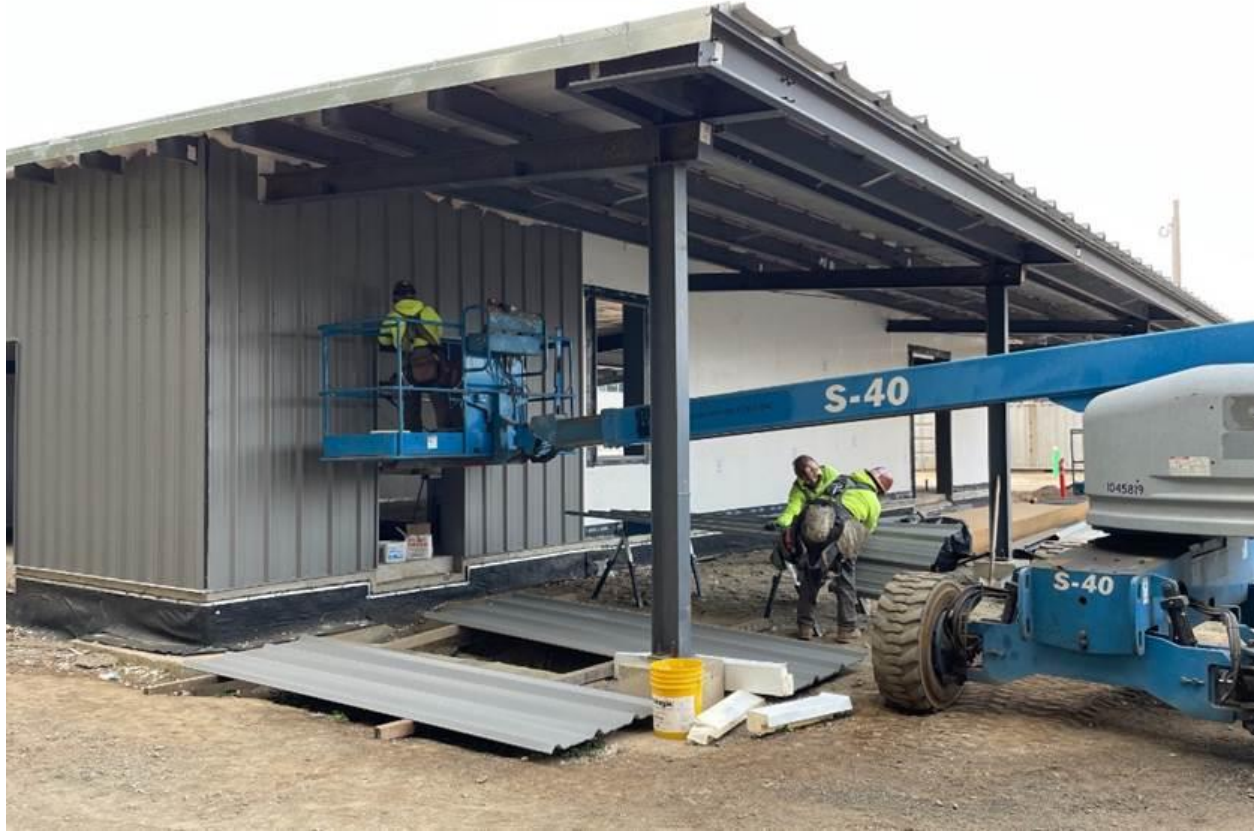
Metal siding installation at the Agriculture Science building
