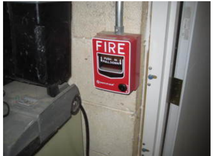
Fire Alarm System Manual Pull Station
