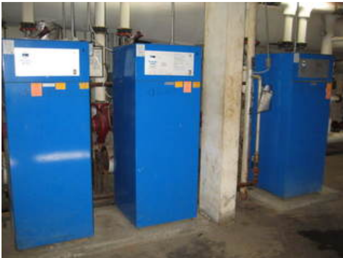
Natural Gas Fired Heated Water Boilers
