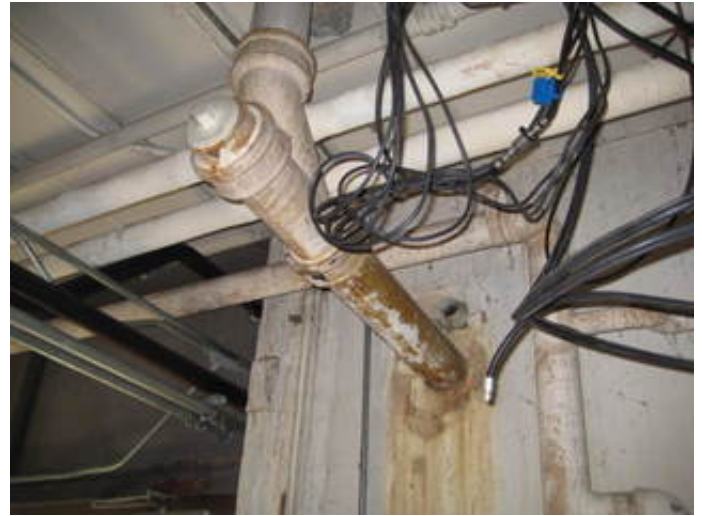
Sanitary Waste Piping
