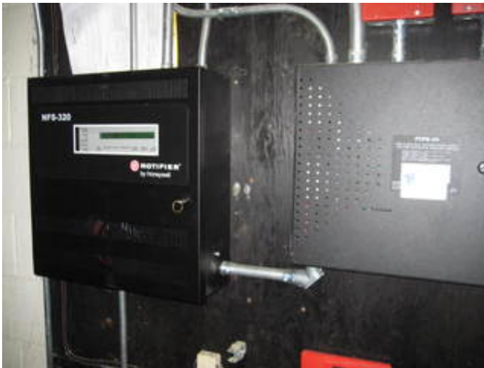
Fire Alarm System Control Panel
