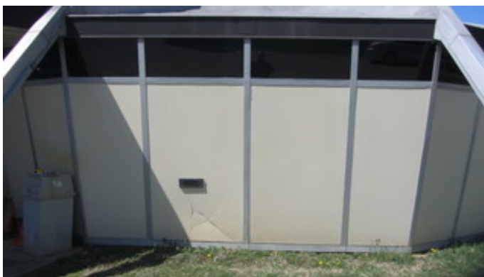
Insulated panels at 1963 Original Construction Music Room
