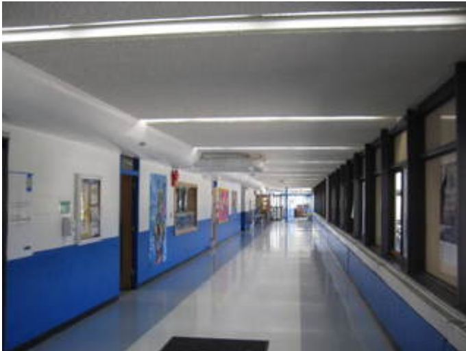
Typical Corridor Fluorescent Light Fixtures
