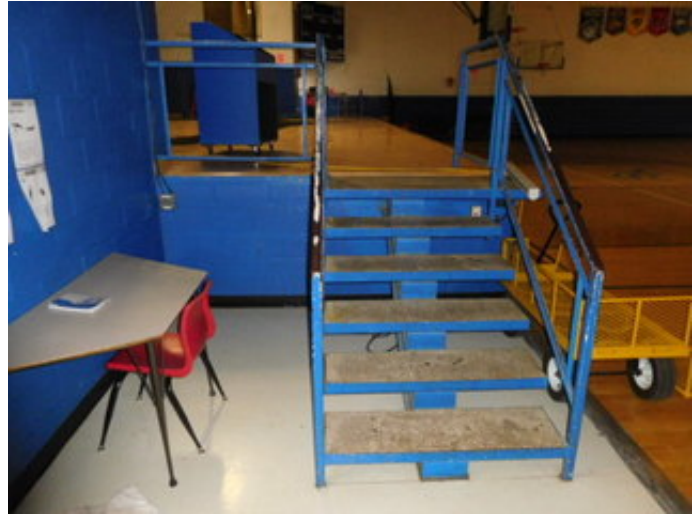
Non-ADA Compliant Stage Access
