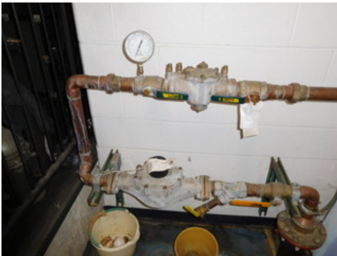
Incoming Domestic Water Service Backflow Preventer
