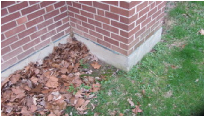
Typical 1952 Original Construction Exposed Foundation
