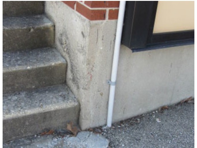
1957 Addition Exposed Concrete Foundation
