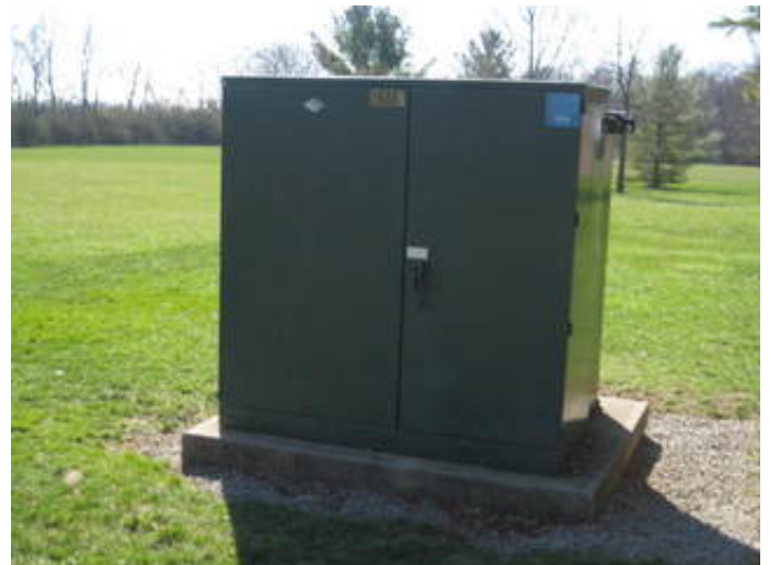
Pad Mounted Transformer
