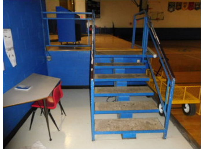
Non-ADA Compliant Stage Access
