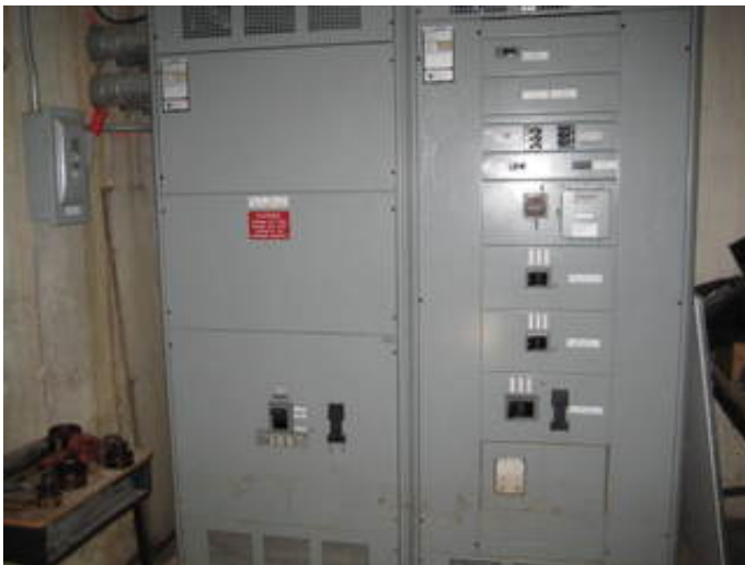
Main Electrical Distribution Panel
