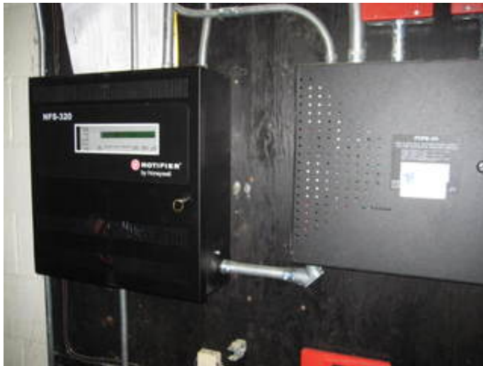
Fire Alarm System Control Panel
