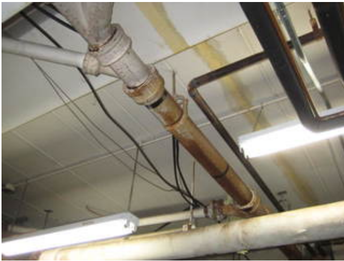
Sanitary Waste Piping
