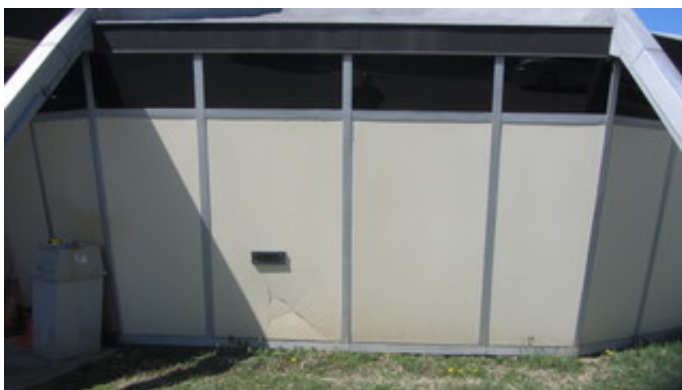
Insulated panels at 1963 Original Construction Music Room
