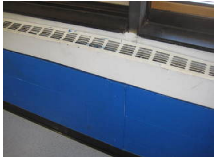
Heating Water Fin Tube Heater
