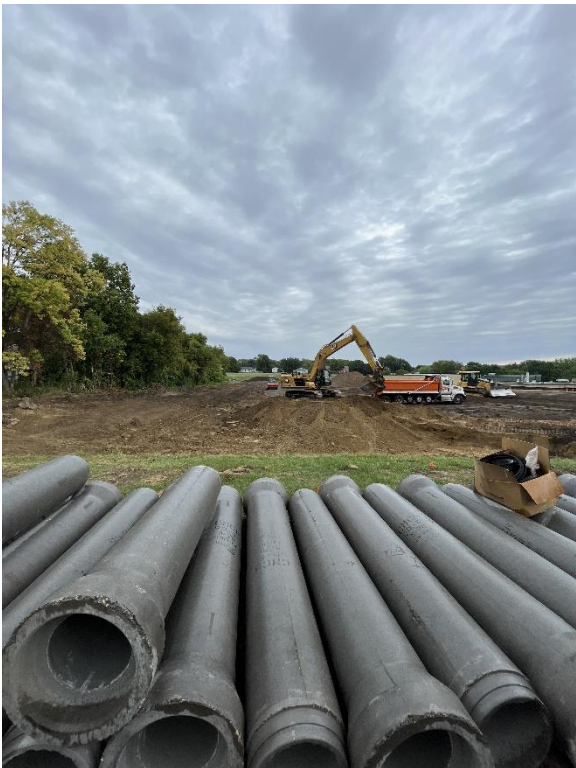
Excavations/Exporting of material for MS retention basin
