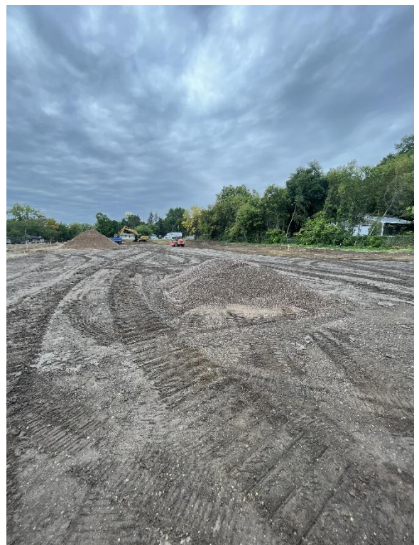
Gravel imported to site after storm sewer and storm structures installed
