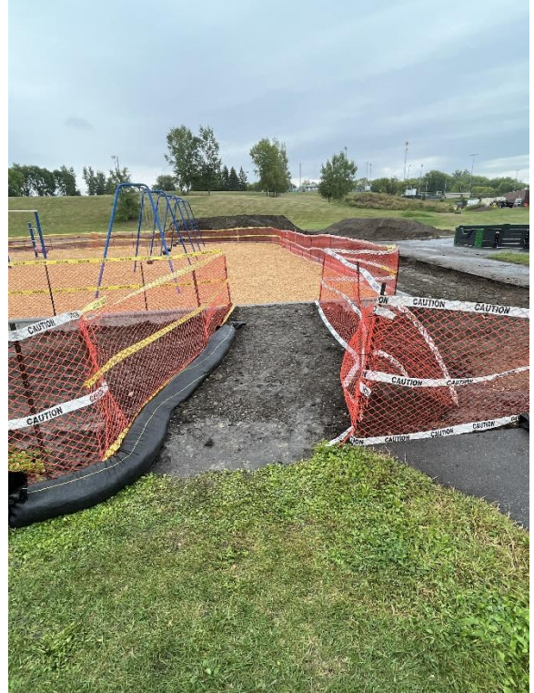
Safety fencing installed keeping active separation between playgrounds and construction
