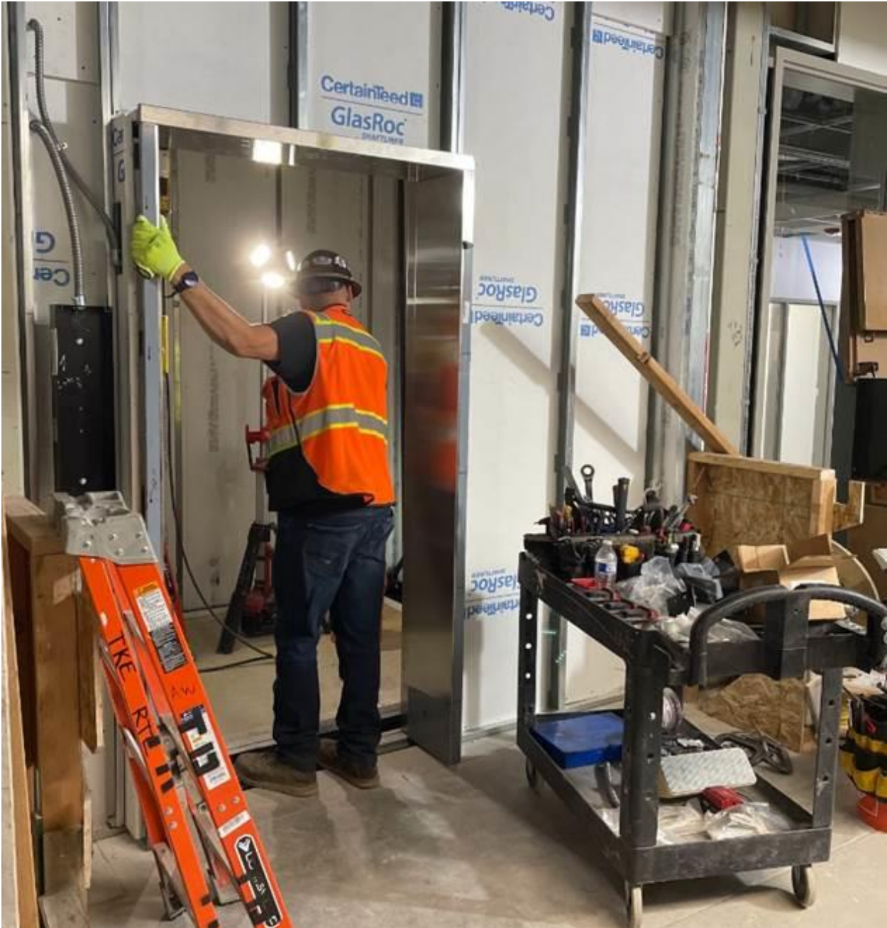
Entryway door and front wall of the elevator being installed
