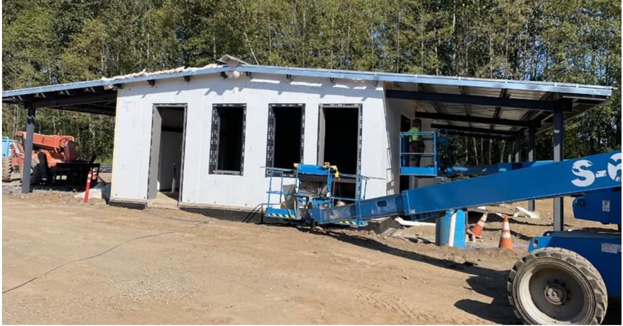
Wall panel installation at the Agriculture Science building
