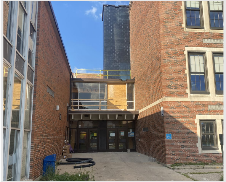
The elevator shaft in the welcome center is built and awaits exterior metal cladding and elevator equipment to be installed later this year
