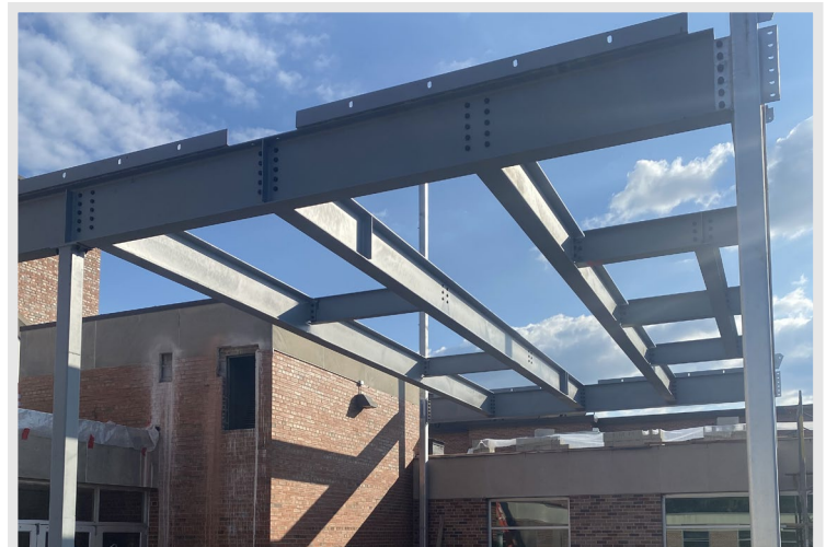
Work will continue during the upcoming school year for the structural steel roof on the new multipurpose room addition
