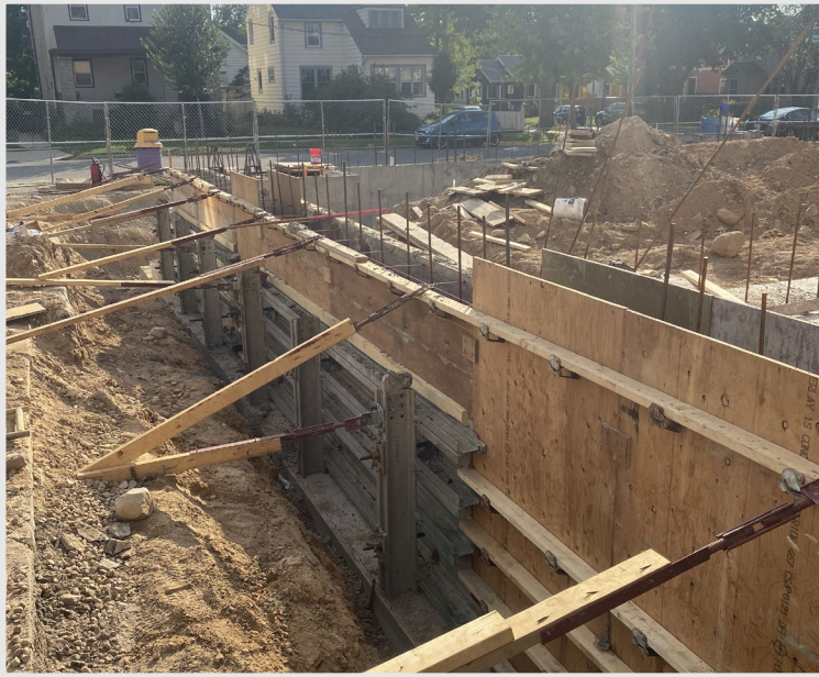
Work on footings and foundations is nearly complete for the new cafeteria and music addition along Fourth Street
