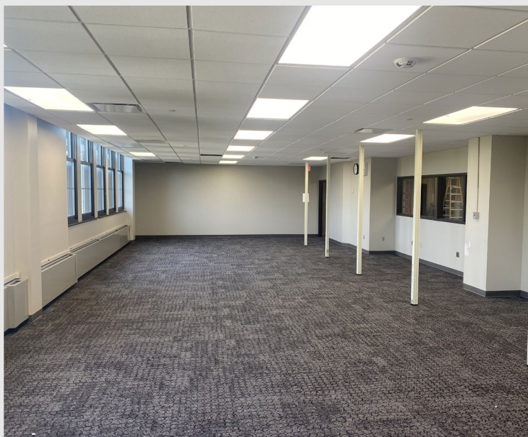
Fresh carpet, LED lights, radiant heat, and wall paint is installed in classrooms on the third floor
