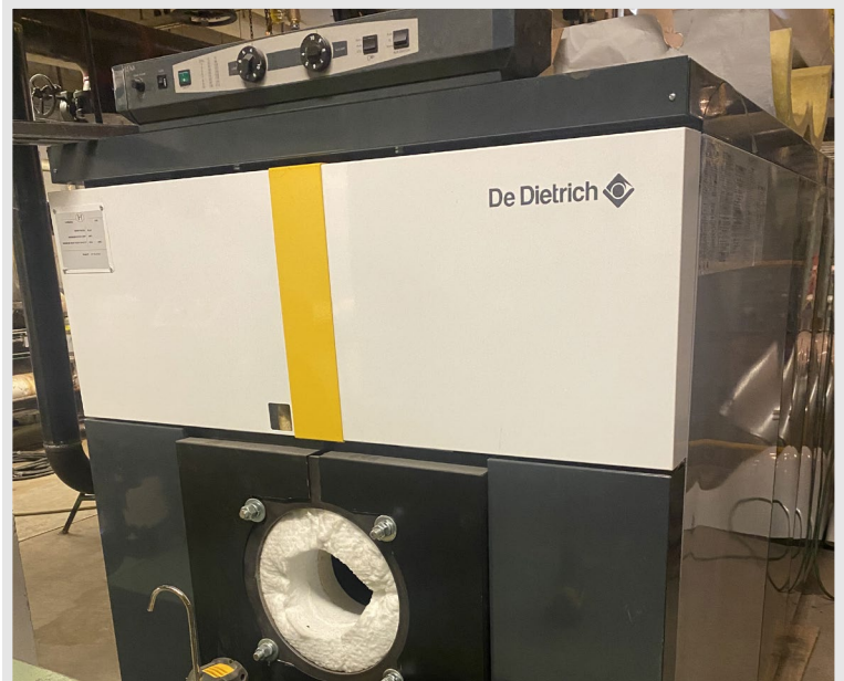
New mechanical boiler equipment is installed and will serve all new hot water infrastructure
