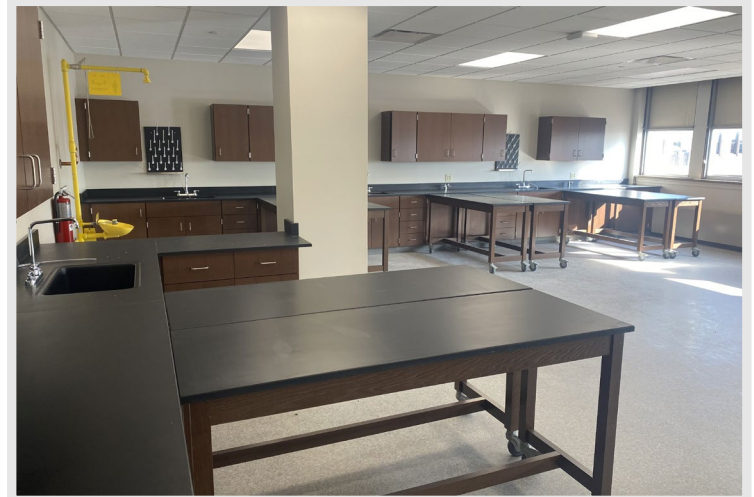
New epoxy lab countertops, casework, flooring, ceilings, and paint are installed in the renovated science lab rooms on the third floor
