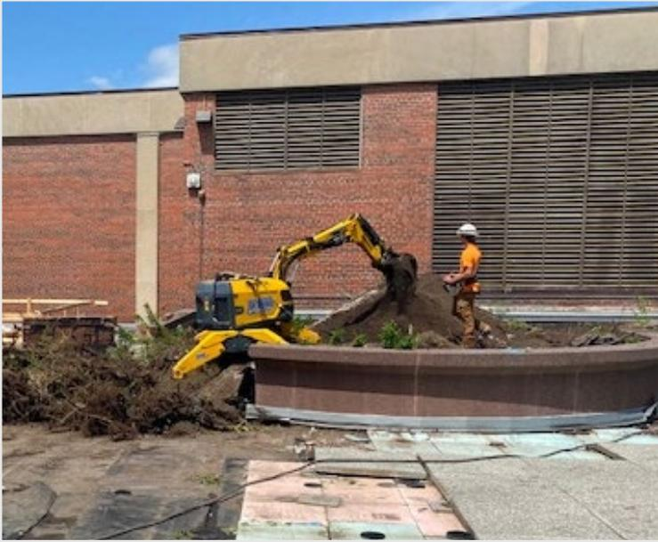
Remote-control robotic equipment is used for demolition work in preparation for the new multipurpose room addition in the courtyard.
