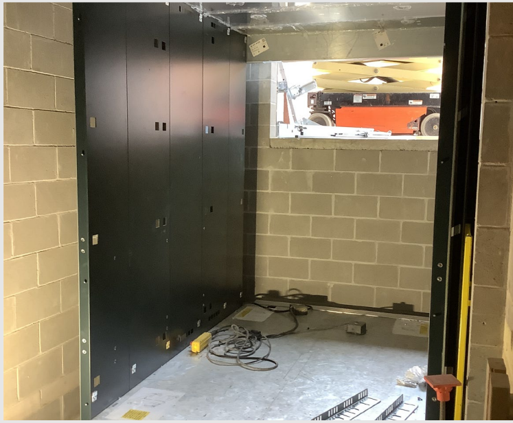
The new elevator is being installed, along with another opening allowing access from the corridor
