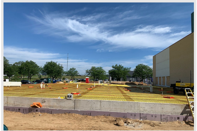
On the south side of the building, work is progressing as the underground utilities, vapor barrier, and concrete reinforcing wire are installed
