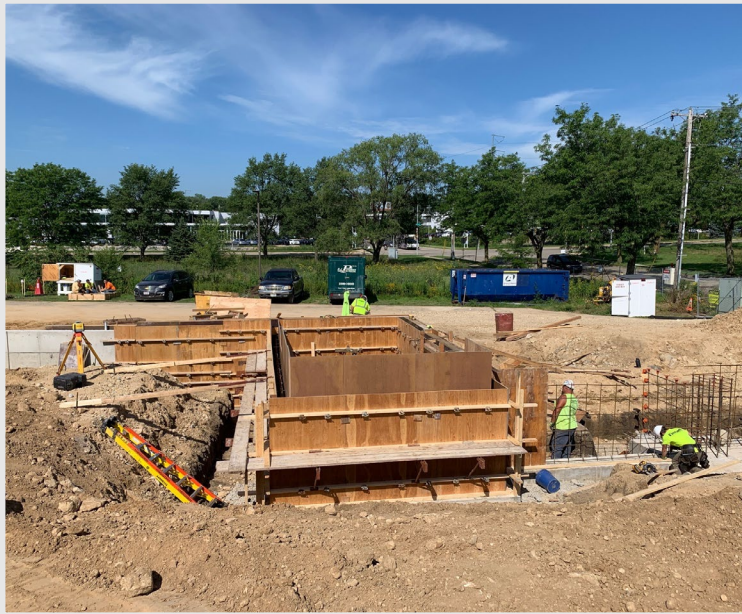
Crews are forming the foundation walls for the west stair tower
