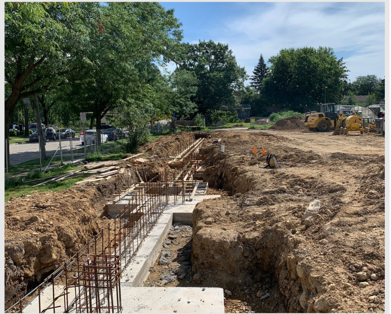
Work is ongoing for the concrete footings on the northwest corner of the site
