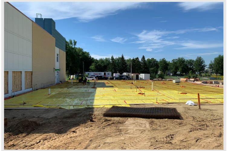
The site is prepped with a vapor barrier prior to pouring the first section of the concrete foundation slab
