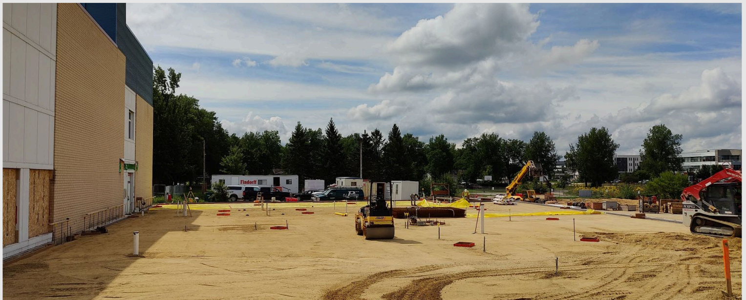
The south side of the site was prepped and leveled in preparation for the concrete foundation pour
