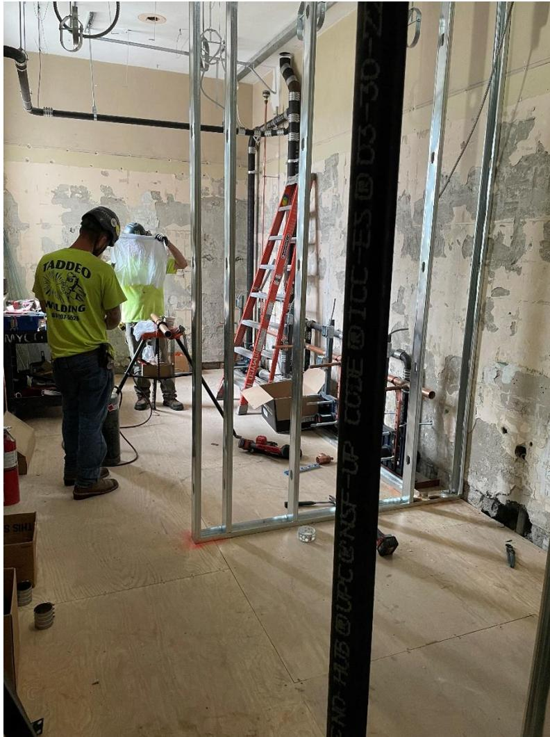
Our bathrooms on the second floor are receiving new walls, flooring, lighting, and plumbing.
