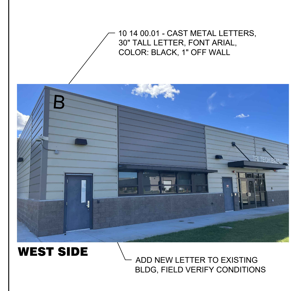
C9 TRI TECH EAST EXISTING BLDG B SCALE: 1/8" = 1'-0"
