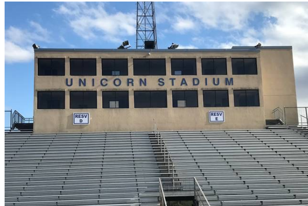
Updating NBHS Pressbox and Providing Artificial Turf to Baseball/Softball
