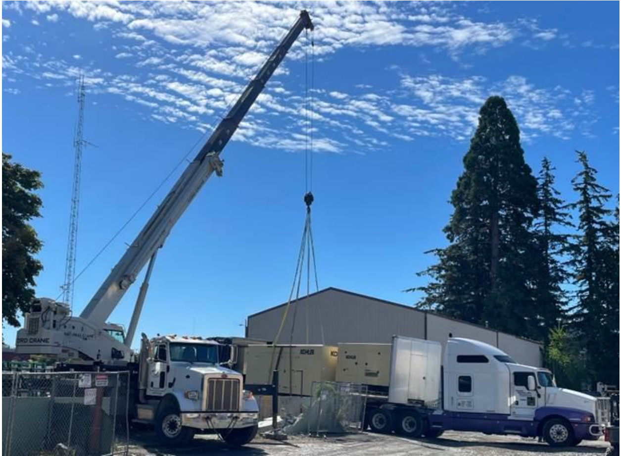
Campus emergency generator being offloaded
