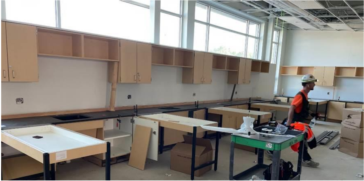
Countertop installation in one of the new science classrooms
