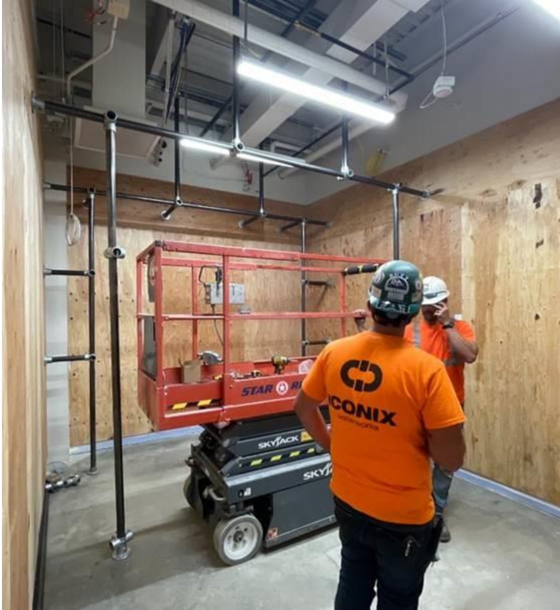
Crews installing the drying rack for football equipment
