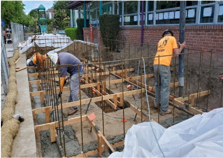
ADA upgrades – ramp in construction
