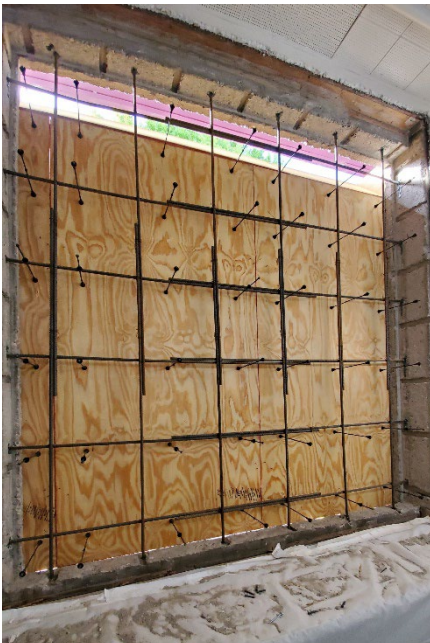
Window structural infill – during construction (required by DSA)
