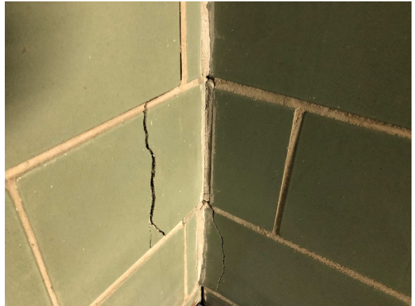
William Ramsay, Stairwell by Rooms 25-30
