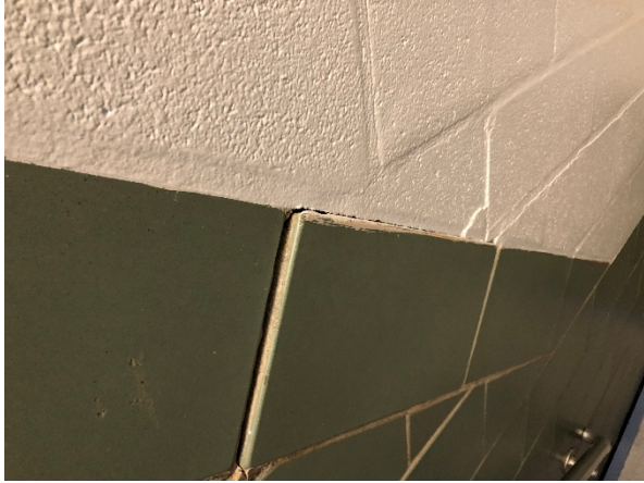
William Ramsay, Stairwell by Rooms 25-30
