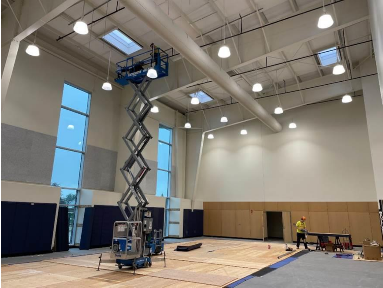
Crews getting started installing batting cages in the P.E. Room
