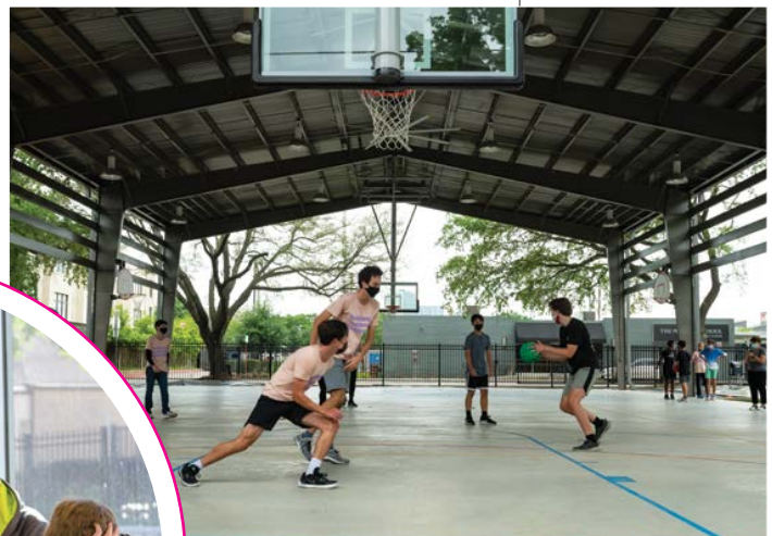
Above: A pavilion was constructed on the South Annex across the street from the Middle and High School, providing an area for sports and more classroom space.
