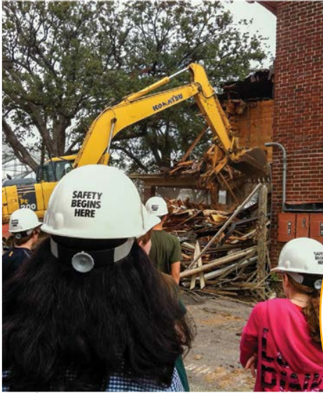
Above: Students watched as an existing structure was demolished at the corner of Autrey and Montrose where the future High School building was built.
