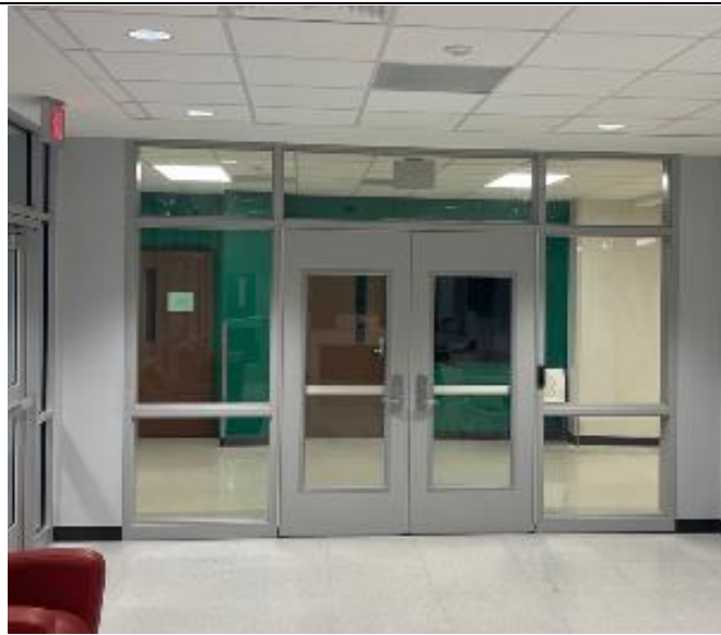
Existing lobby door with card reader.
