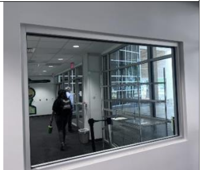
Security office window glazing.
