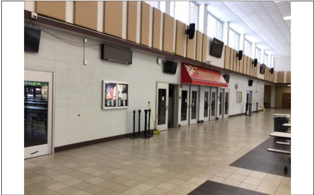
Kitchen doors have been installed.
