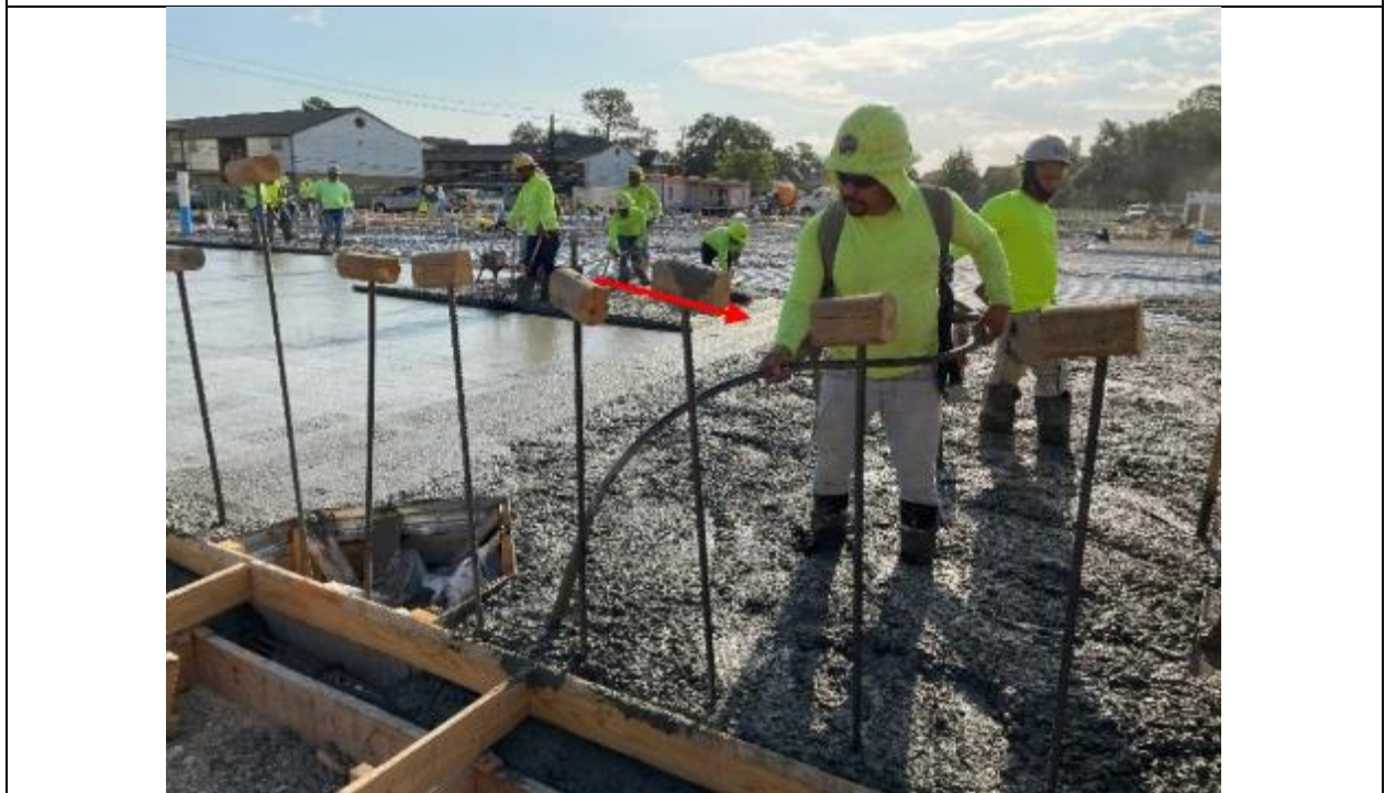
Concrete vibrator to avoid air pockets
