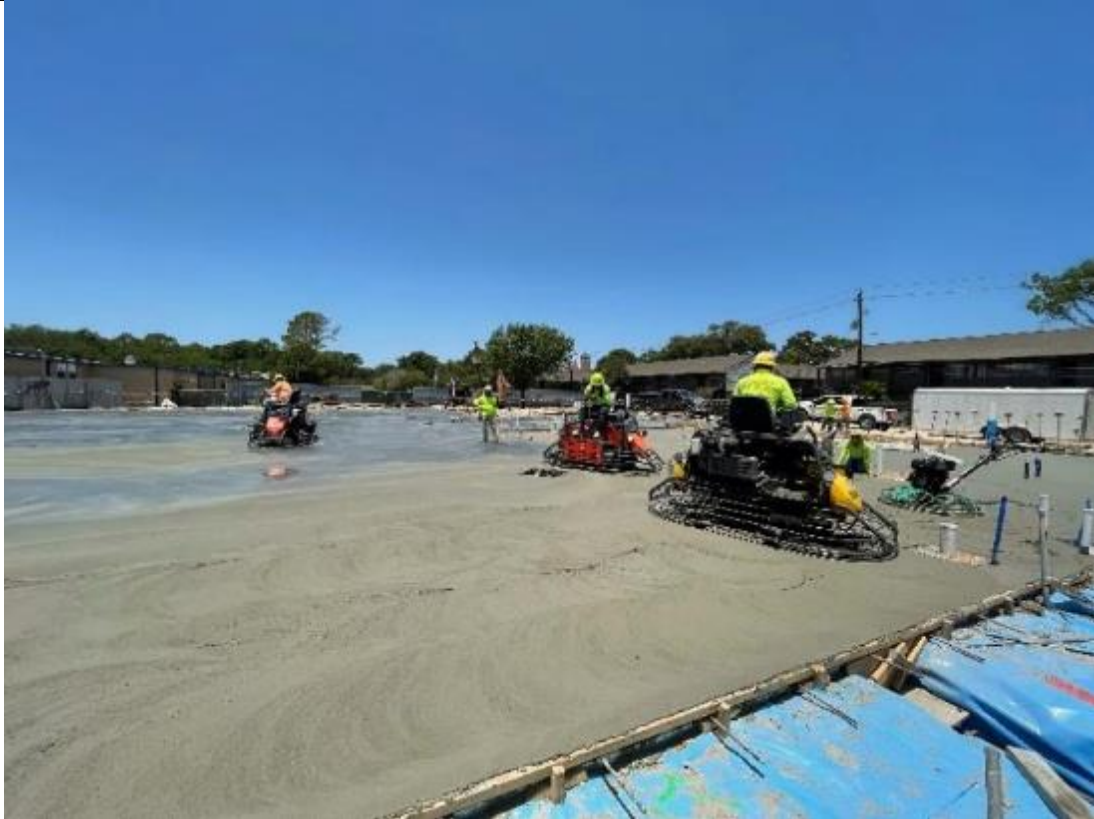
Power trawlers stabilizing and smoothing slab
