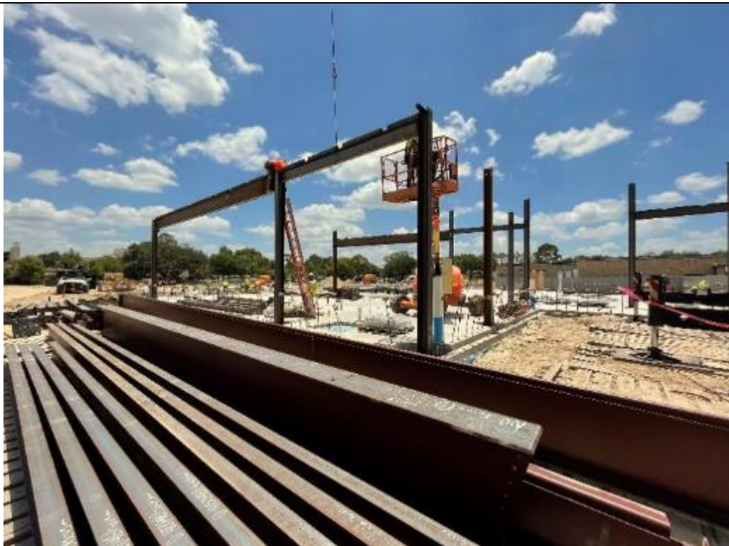
Steel. Area D
