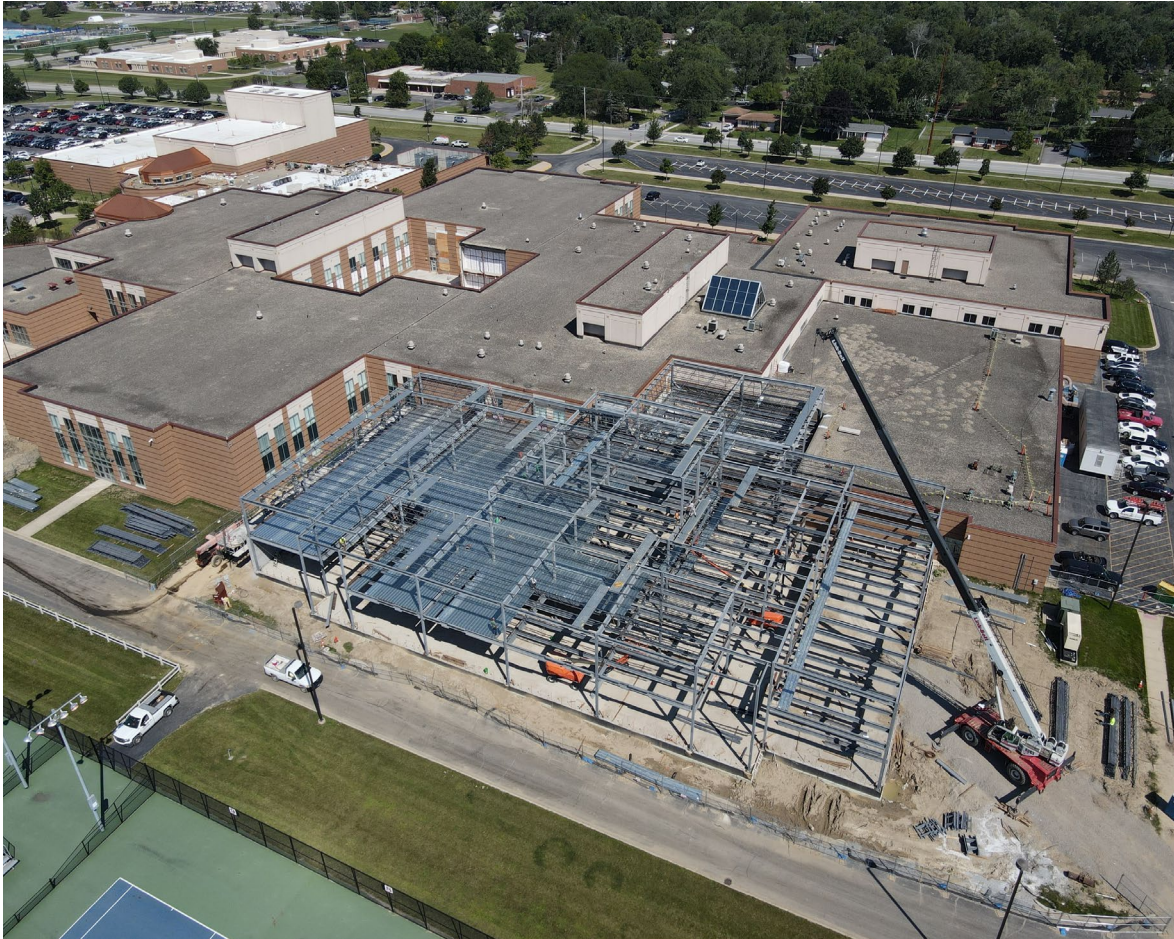
Classroom Addition Structural Steel
