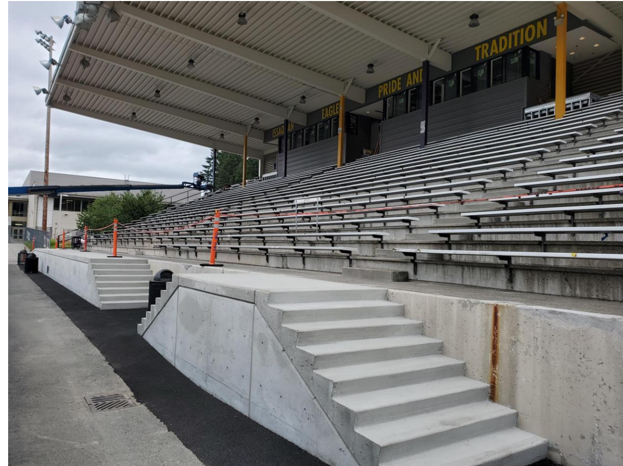
New ADA accessible ramp and stairs installed
