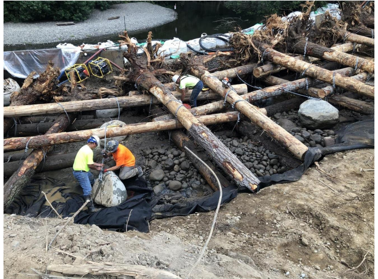
View of coffer dam and "fish friendly" creek bank repairs
