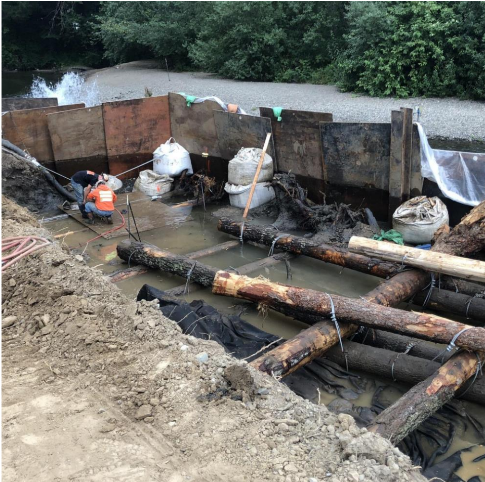
View of coffer dam and "fish friendly" creek bank repairs
