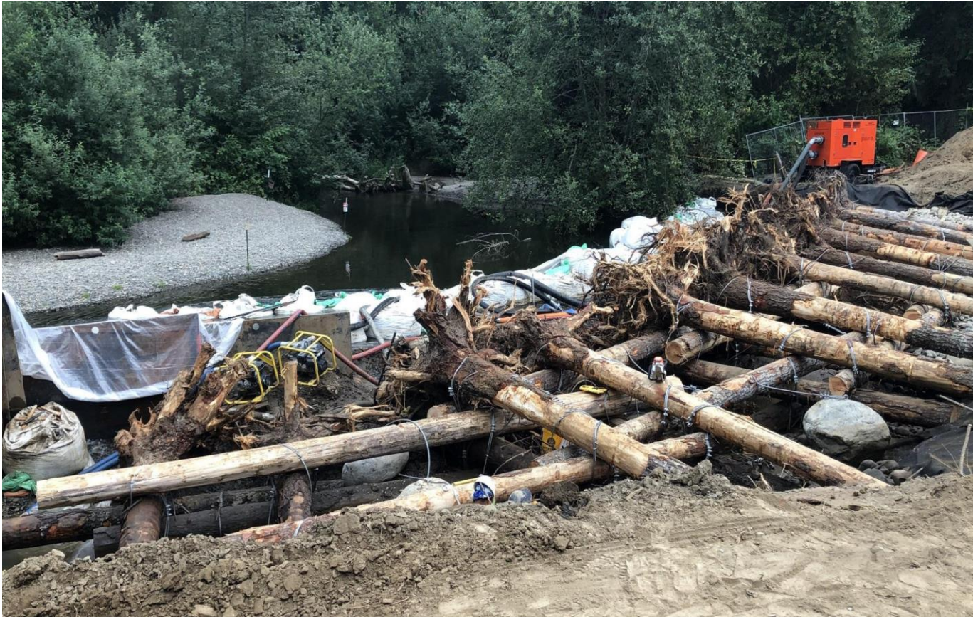
View of coffer dam and “fish friendly” creek bank repairs
