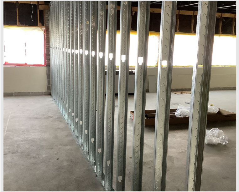
Walls in the new classroom spaces are being framed
