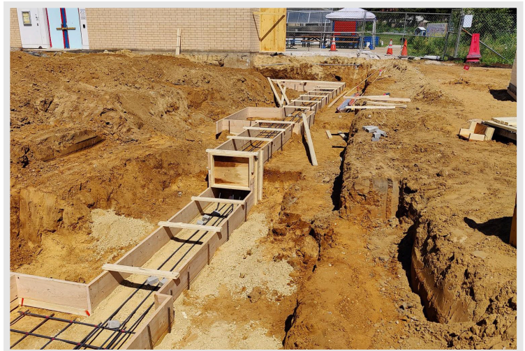
Strip footings were installed in preparation for the concrete to be poured
