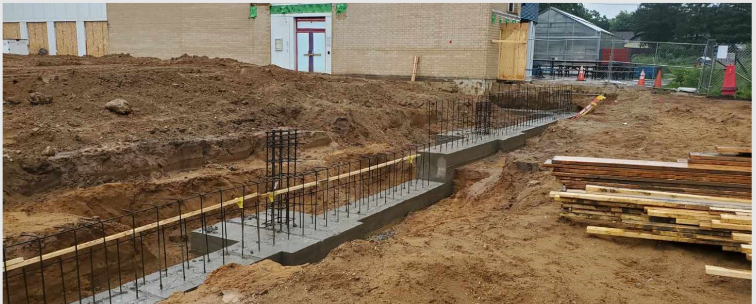
Concrete footings on the south end of the building are complete
