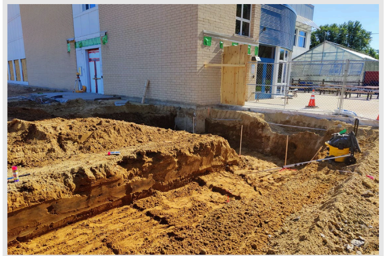
Excavation work started for the building's footings and foundation
