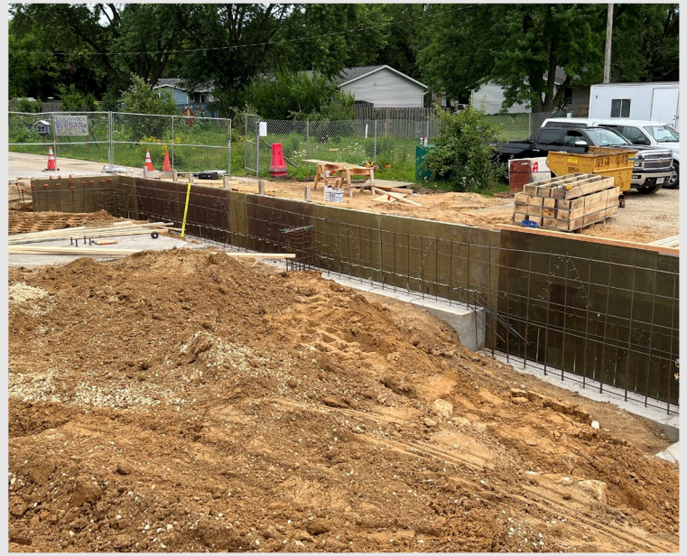
The building's foundation walls have started to take shape
