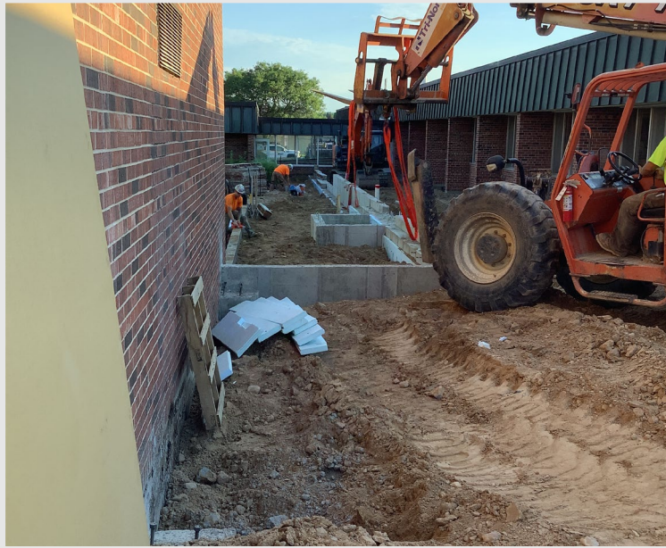
The concrete foundations for the courtyard expansion are ready to be backfilled, which improve building circulation when complete
