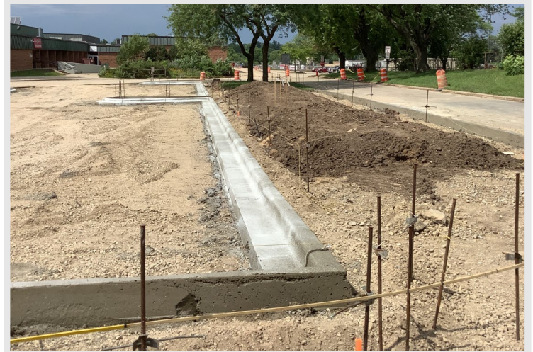
The new concrete curb for the south parking lot and entrance has been poured
