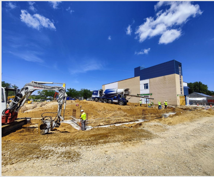
Construction crews poured concrete for the building's footings
