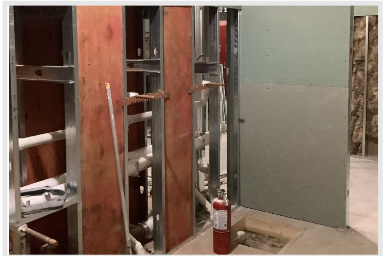
The bathroom walls were framed, and in-wall support blocking and drywall are being installed
