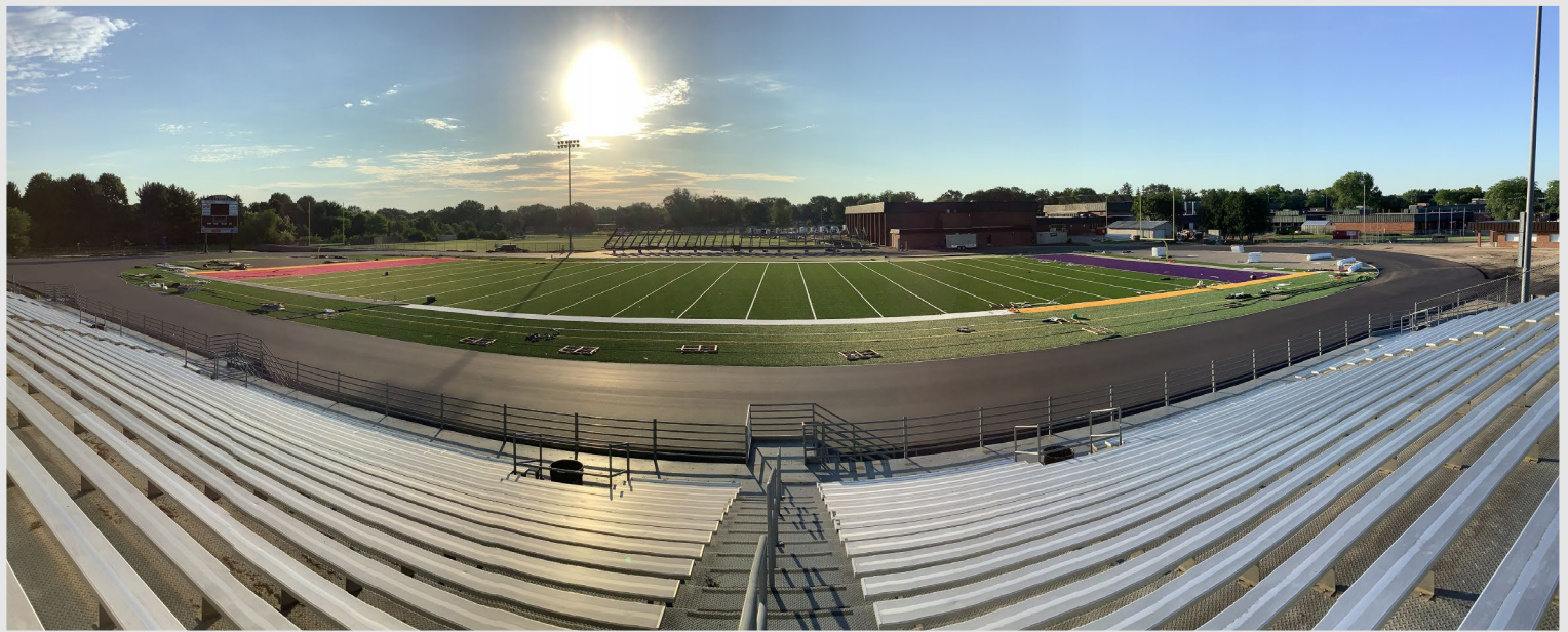
Crews made significant progress on Lussier Stadium with a new turf field, track, and bleachers
