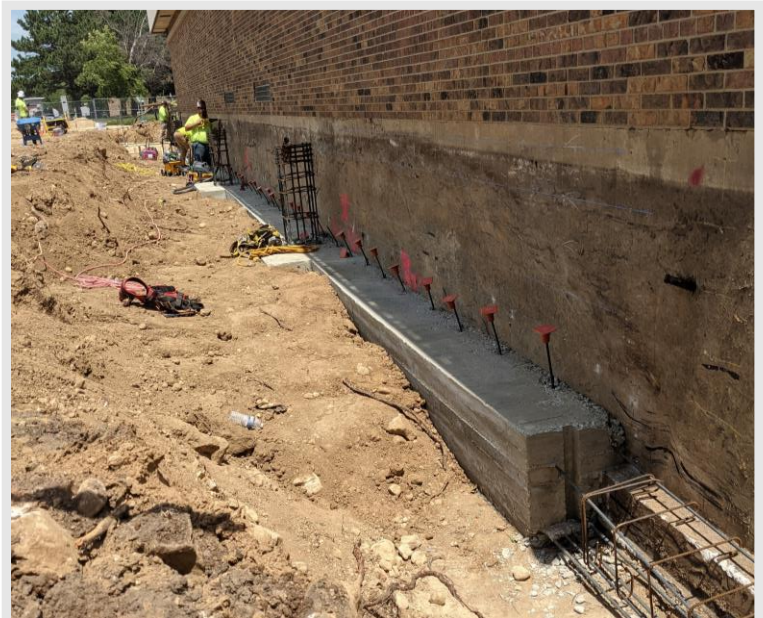
Iron workers are installing rebar to support the new structural steel columns in the new music addition foundation
