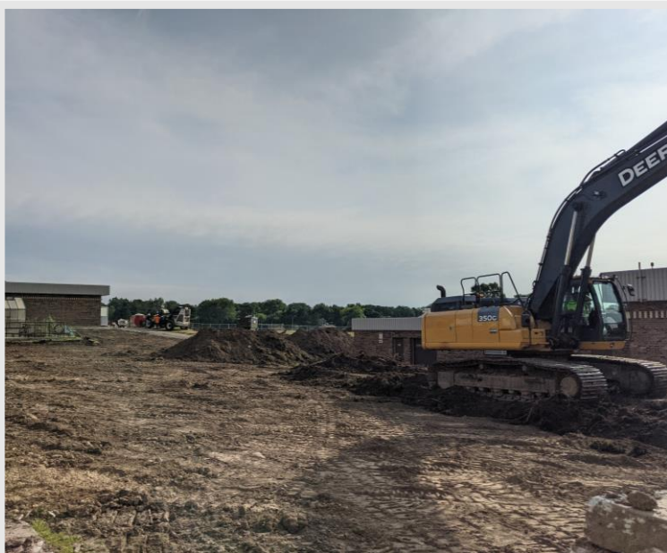
Crews have started preparing the soil for the applied technology wing expansion
