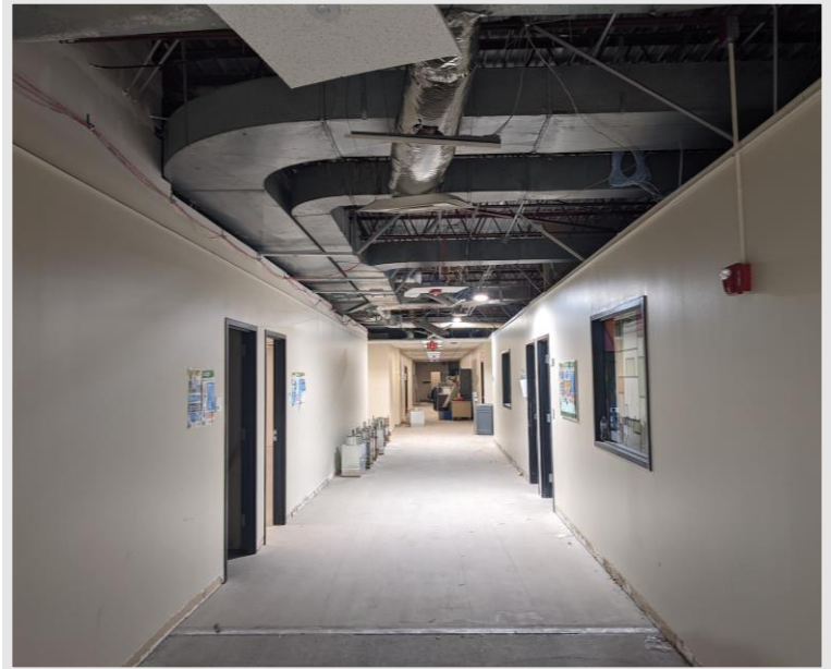
Ceilings have been removed and duct work is being replaced throughout the building to improve air flow
