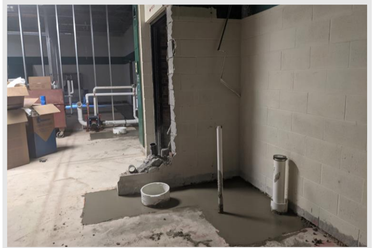
Underground plumbing work in the restrooms is complete and the concrete slab has been laid
