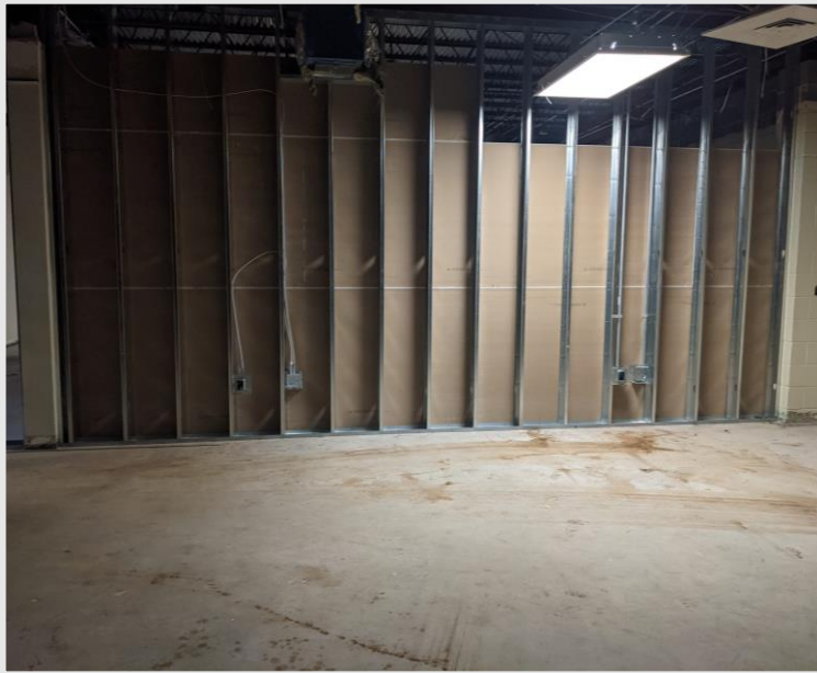
New steel stud walls are replacing temporary partitions throughout the school, which will reduce noise in learning spaces
