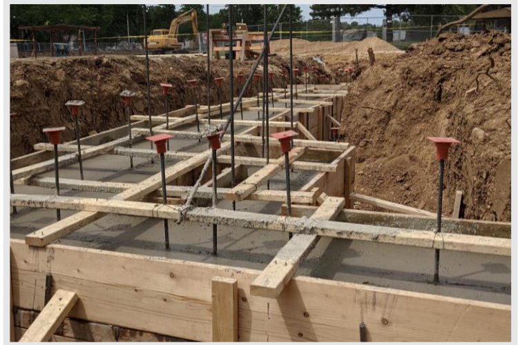
Concrete was poured for the footings and foundation of the new music addition
