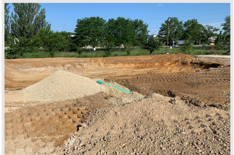
Workers constructed a stormwater retention basin on the construction site
