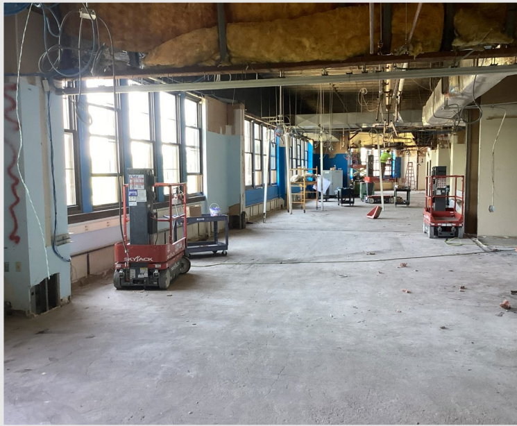
Mechanical, engineering, and fire protection systems are beginning in the third floor classroom renovation area
