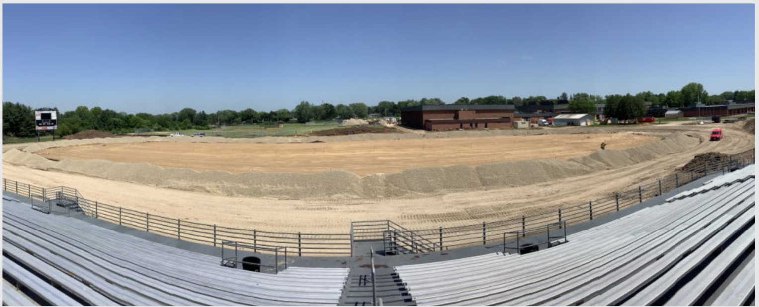
The stadium area is being prepped for the curb that will go around the track
