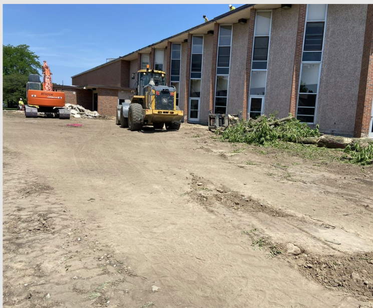
Workers are preparing the site for the cafeteria and classroom additions
