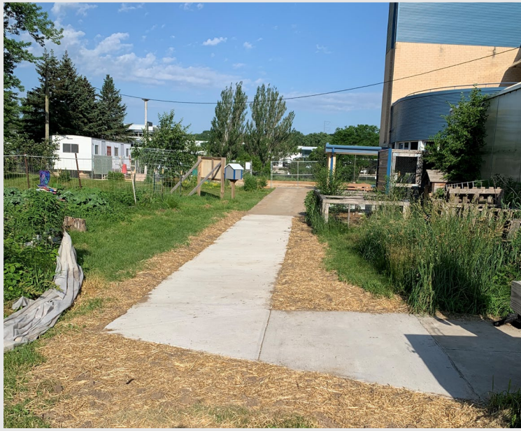
A temporary sidewalk was added as a new access path to the rear entrance of the Badger Rock building
