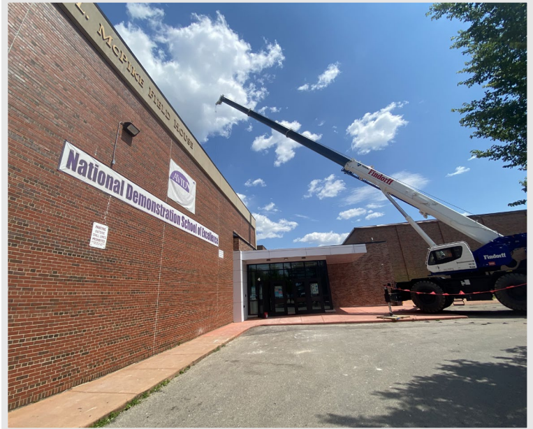
Construction equipment is used to move demolition debris from the locker room renovation area
