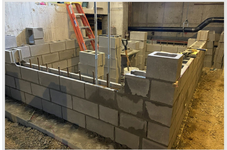
The walls for the new welcome center elevator shaft are being built
