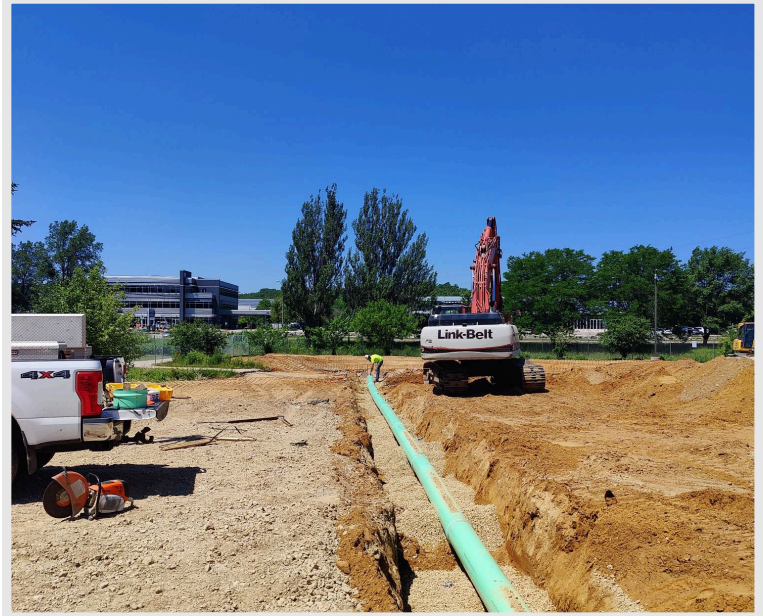
Crews installed stormwater piping, which will drain water into the stormwater retention basin
