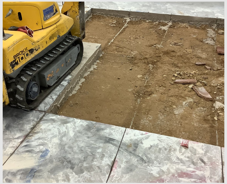
Concrete has been cut and the new elevator pit is being excavated
