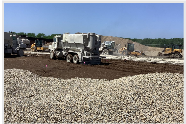
Workers are wrapping up soil stabilization work in the stadium area
