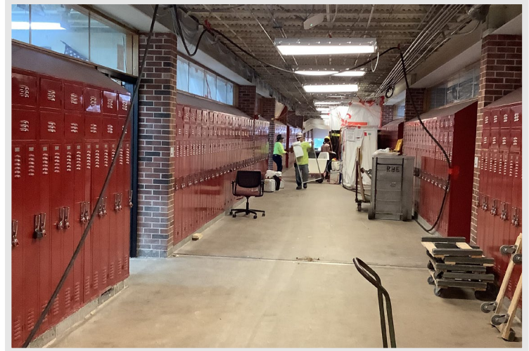
Demolition is ongoing in the classrooms and hallways in preparation for new finishes
