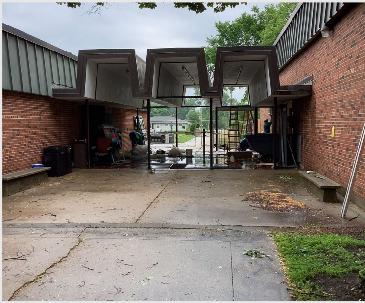
Demolition is progressing in the breezeway with the removal of the existing glass and doors
