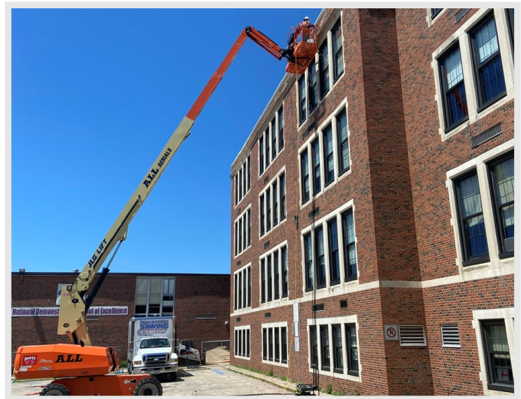
Masonry restoration work is ongoing throughout the existing façade to protect the building's historic architecture
