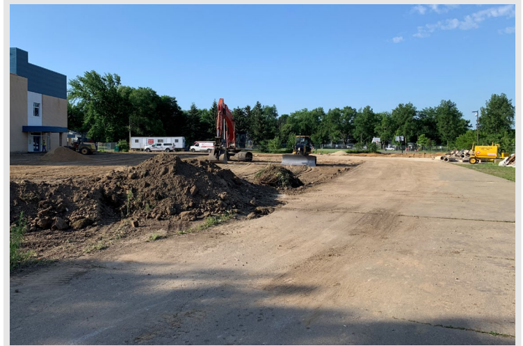
Construction equipment and trailers are on the Badger Rock site starting work on the new Southside Elementary School
