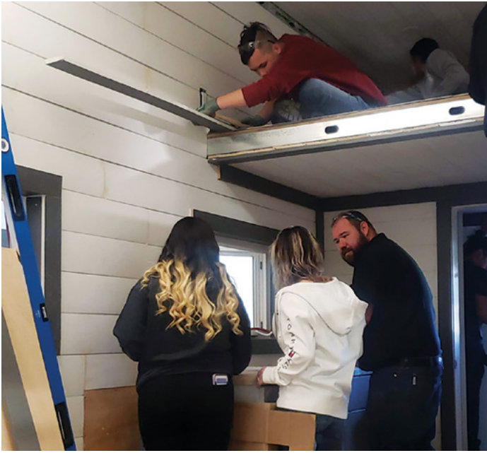
Construction students working on the inside of the tiny house.
