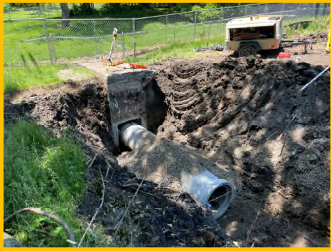
Continued Storm Sewer Install
