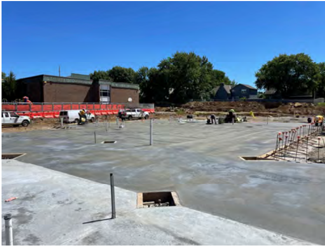
Section 3 Slab on Grade Poured
