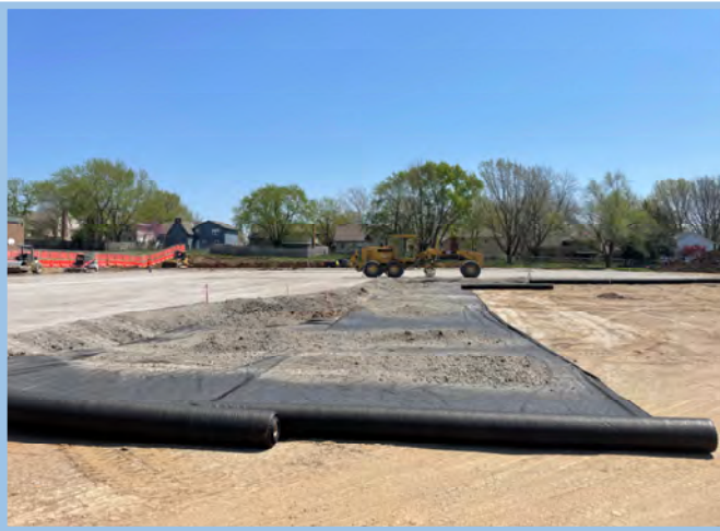
Laydown Filter Fabric
