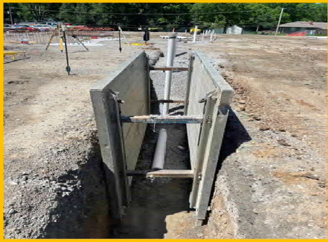
Plumbing Underground Sanitary
