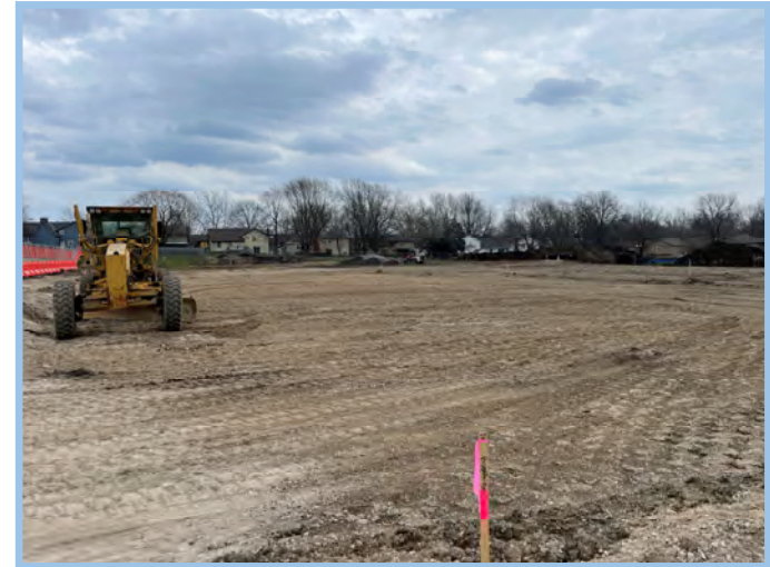
Compaction of Building Pad
