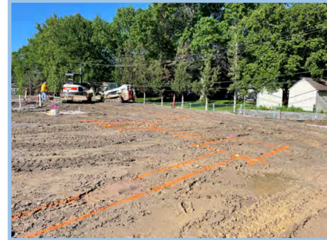
Continued Footing Layout and Excavation
