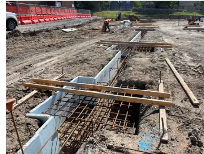
Continued Footing Formwork & Prep
