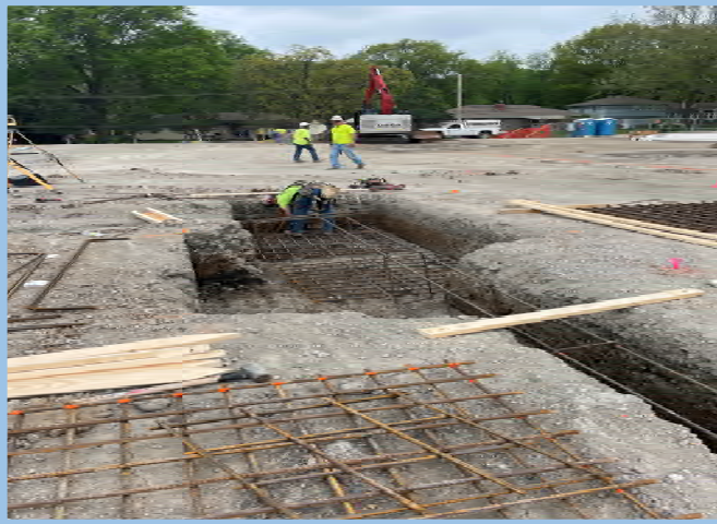
Footing Reinforcement Install
