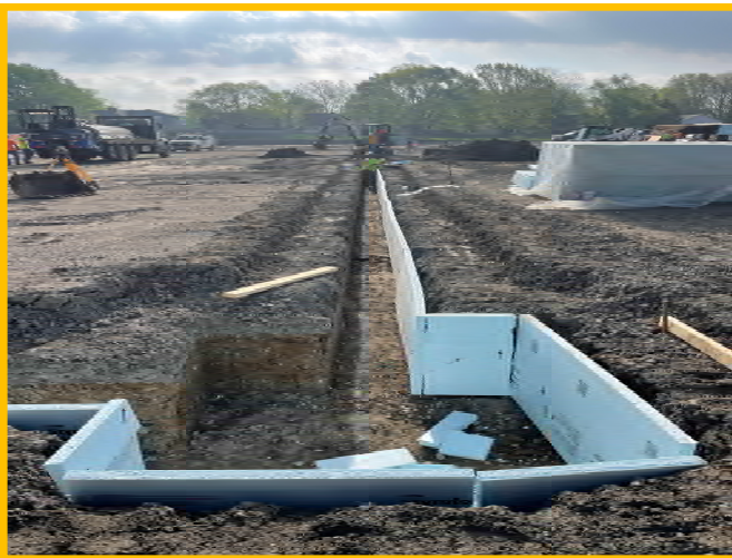
Foam Board Install
