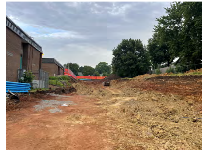
East Side Backfilled to Grade
