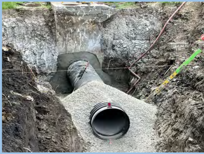
Storm Sewer Install
