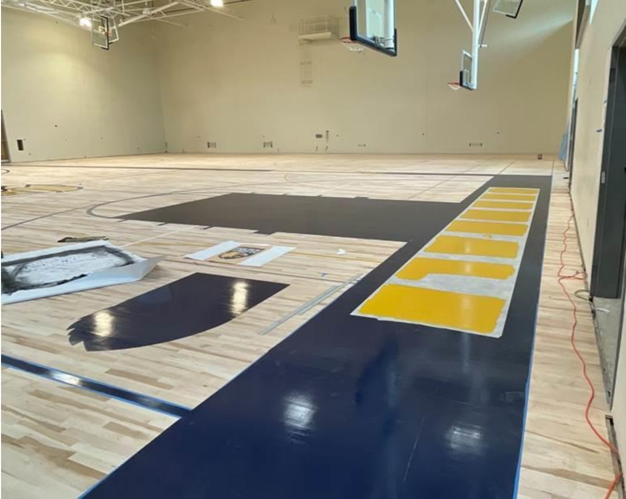
Gym floor striping process
