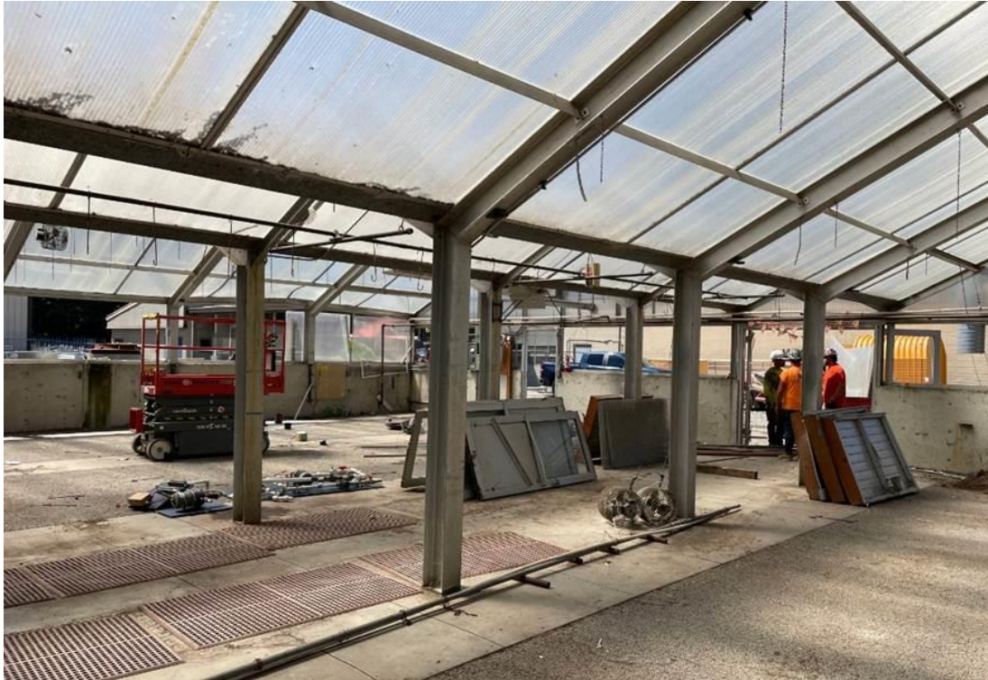
The beginning of the Greenhouse framework disassembly
