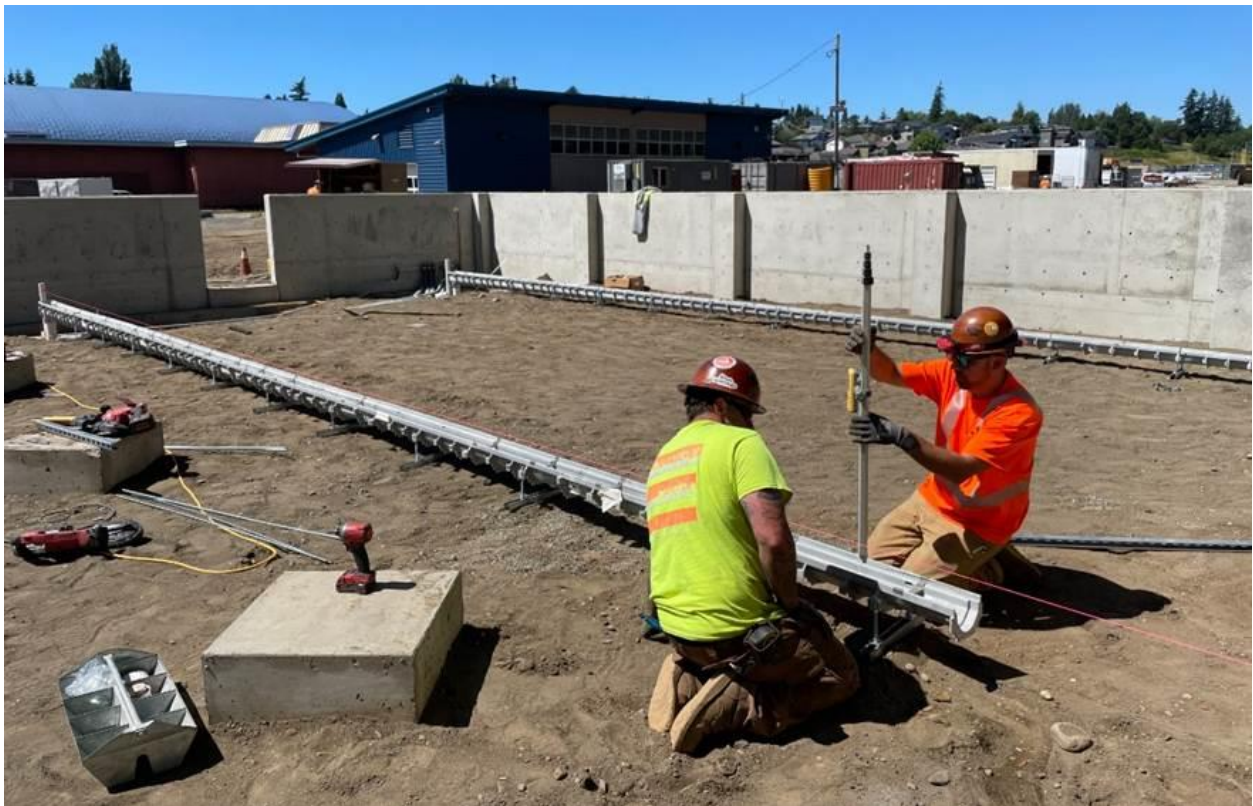
Crew installing the trench drains in the new Greenhouse
