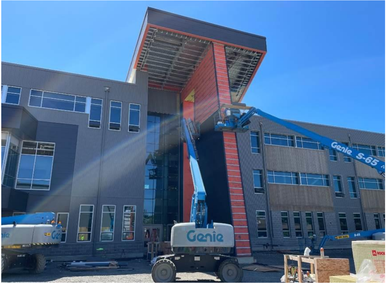
Final siding at the new main entry is underway
