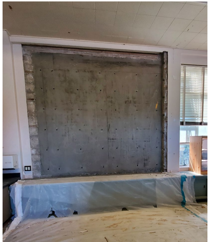
New concrete panel placed at existing window opening
