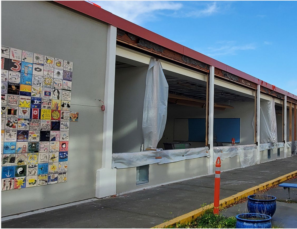
400 Building – Prepping for window installation
