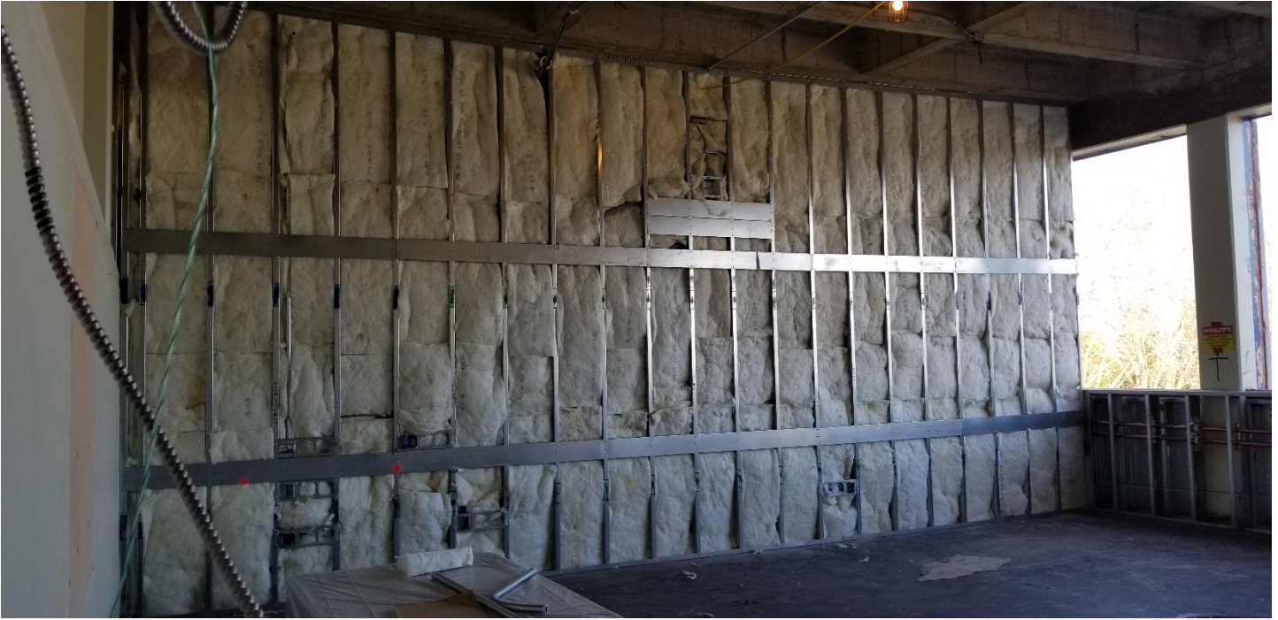
200 Building – Metal framing and insulation installation in typical classroom under construction
