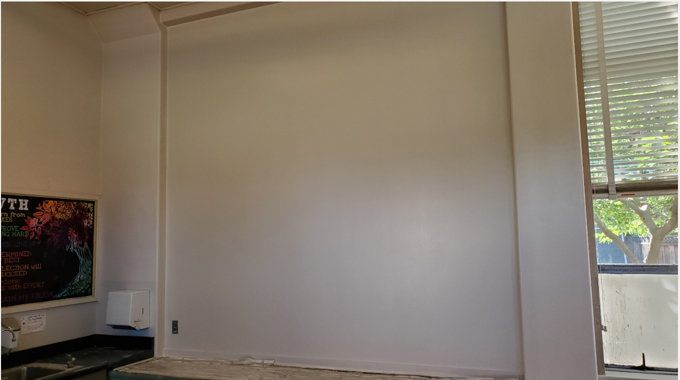
Finished paint coat at new wall placed window infill (interior)
