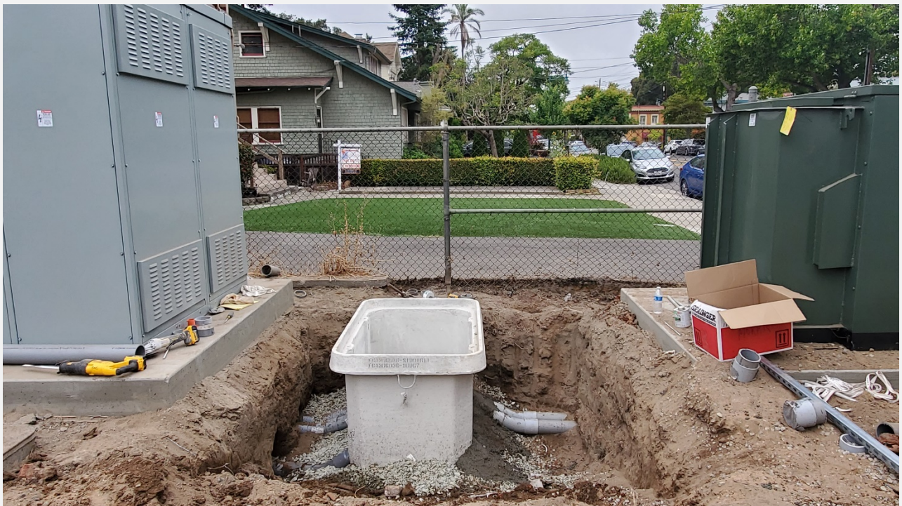
New transformer pull box
