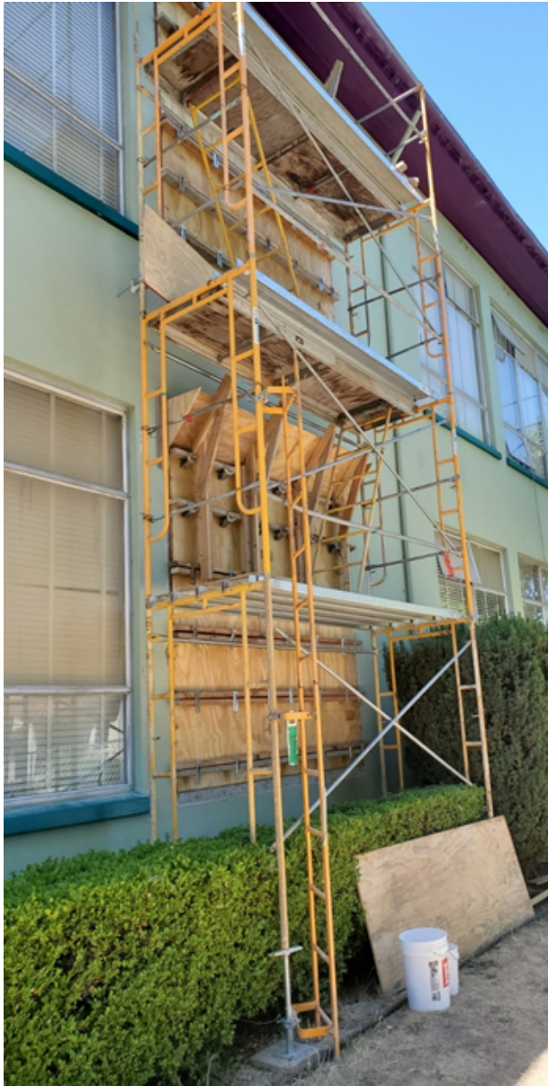
Building A – Window demo for concrete infill to meet structural requirements from DSA and bring the building up to structural code
