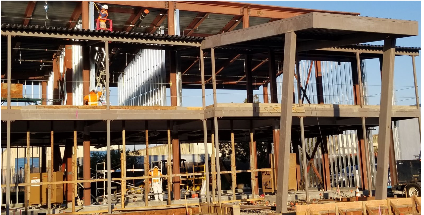
Building 900 – Framing of one of two stairways accessing second floor
