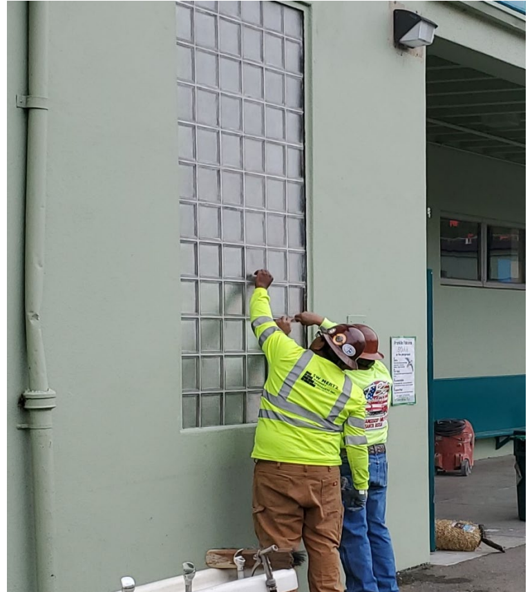
Glass block window – removal of existing caulking
