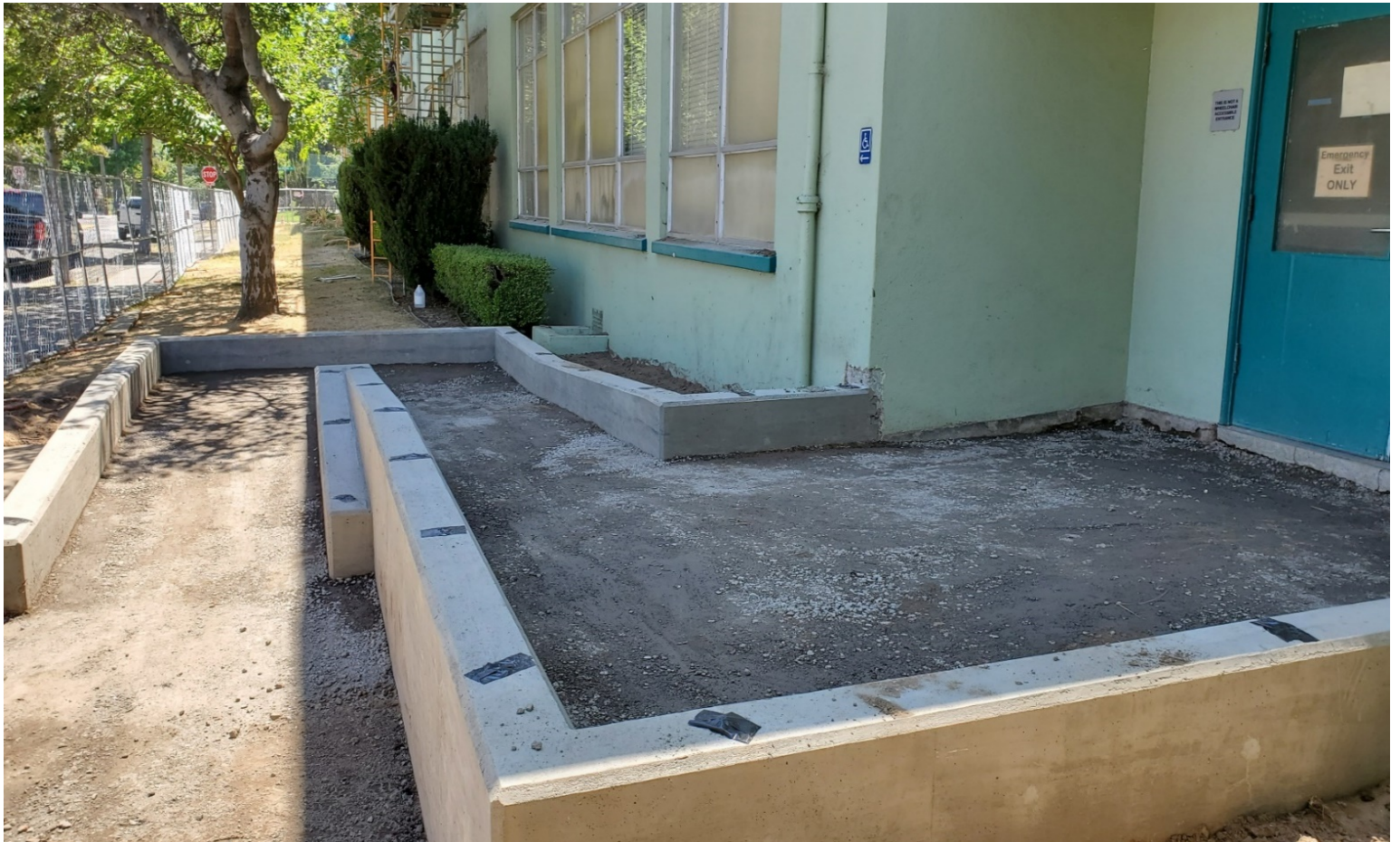
Concrete and wall placed at new ADA ramp
