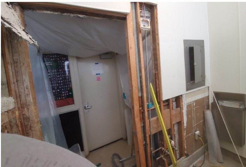
Existing toilet room wall and door opening demo
