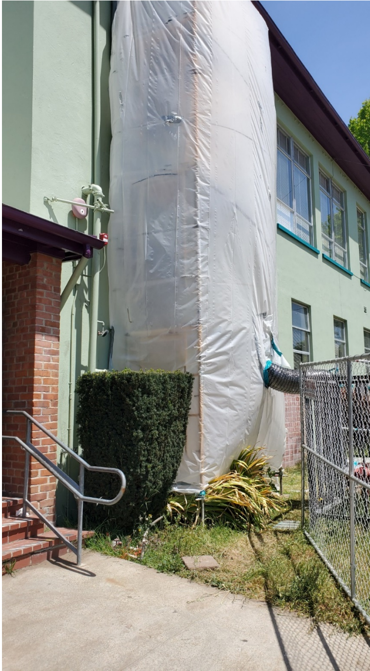
Glass block repair due to water intrusion. Typical for all glass block windows throughout the school.
