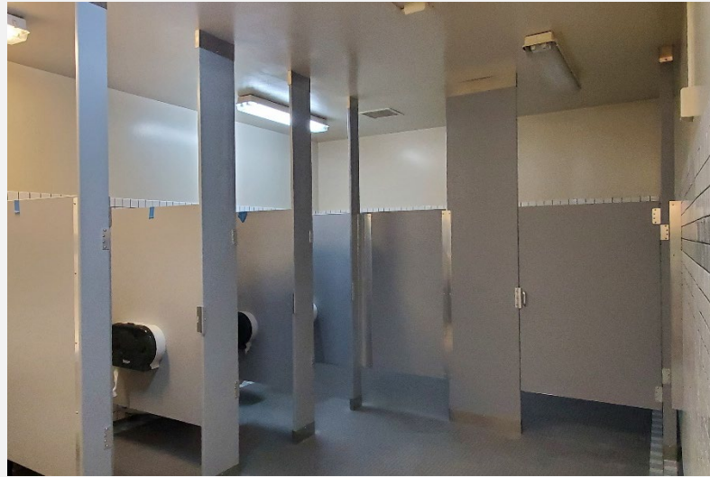
New partitions installed in toilet room
