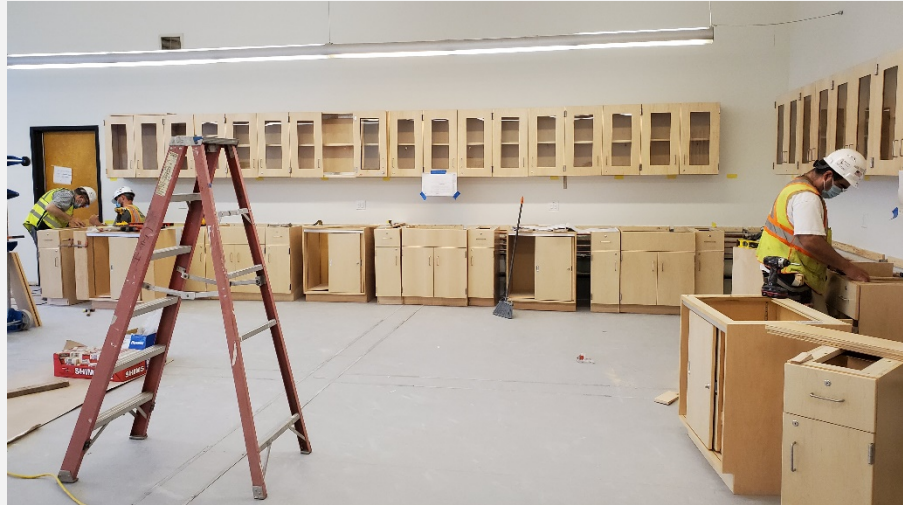
100 Building - Cabinet installation in science classroom
