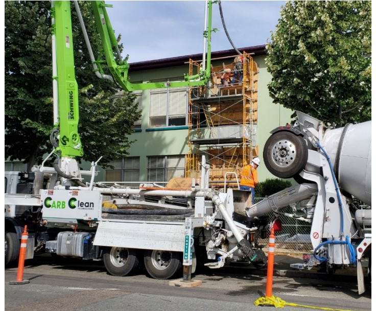
Building A – Concrete infill at existing window opening
