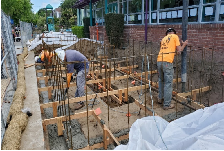
Footings and reinforced steel for ADA ramp
