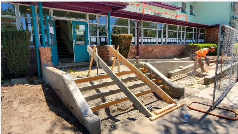
ADA accessible ramp installed at school entrance
