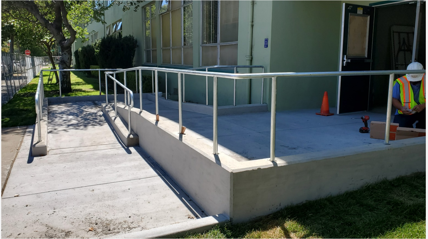
ADA accessible ramp installed at school entrance
