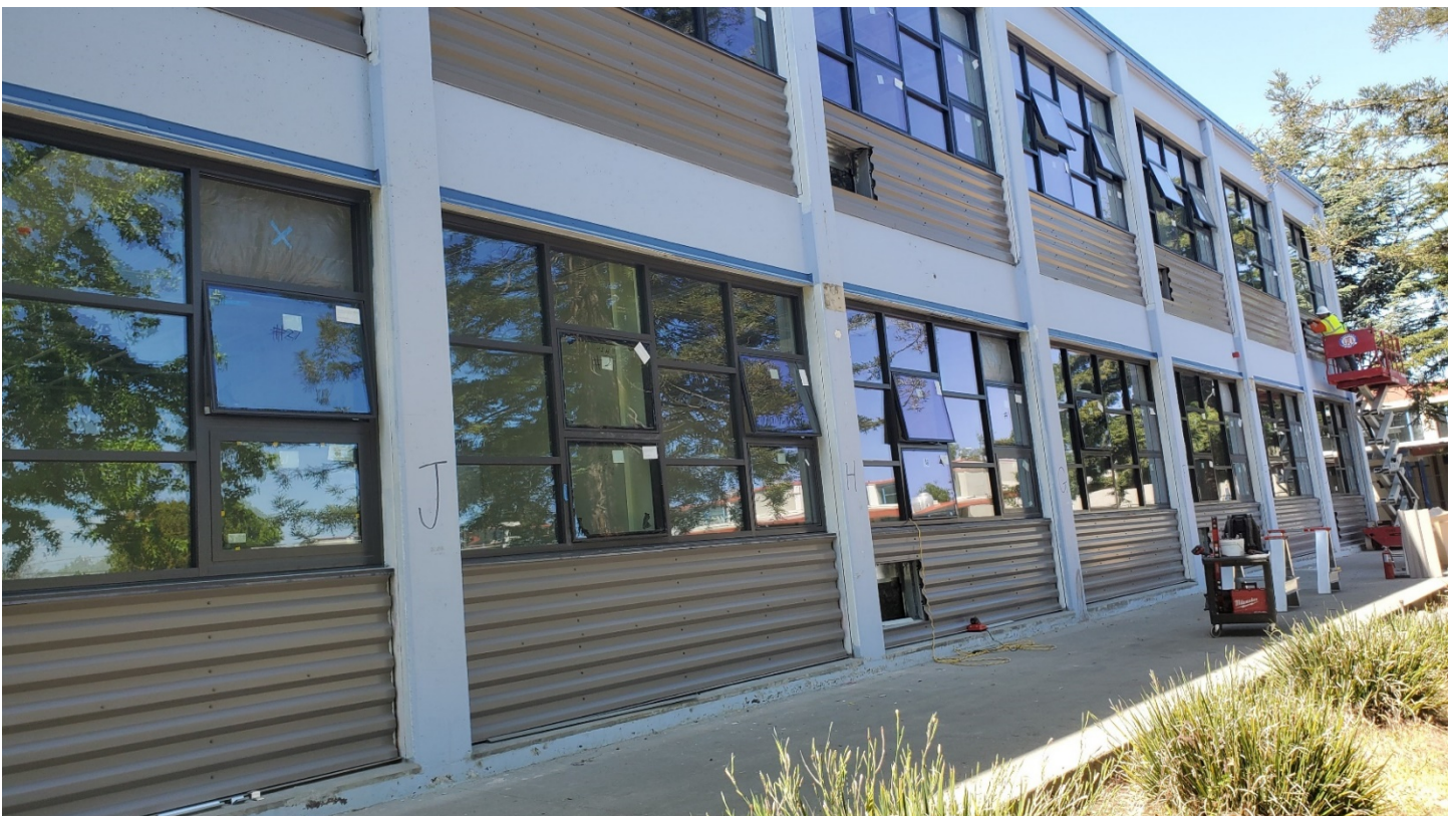
200 Building – Window installation in progress
