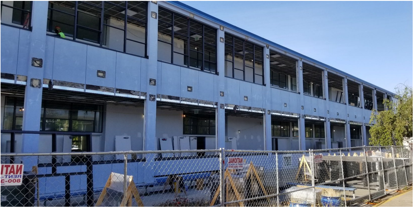
200 Building – Start of window framing
