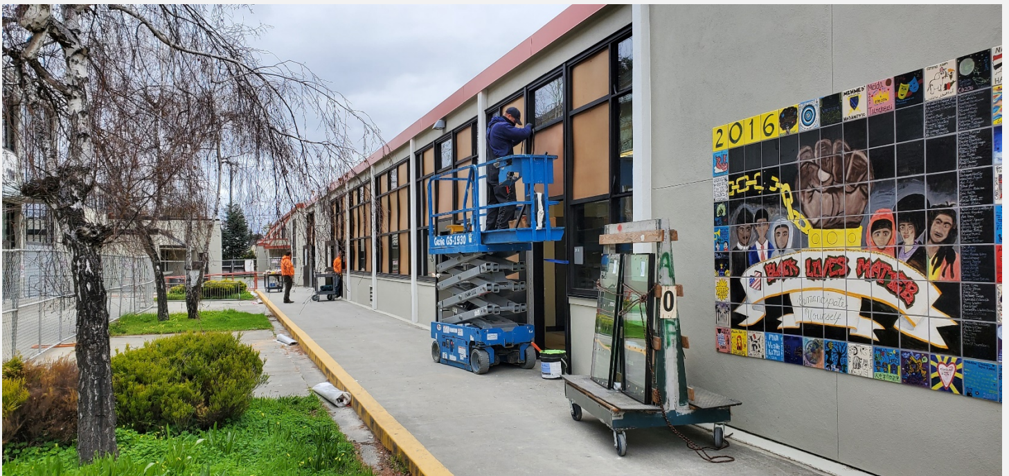
300 Building – Storefront windows installed
