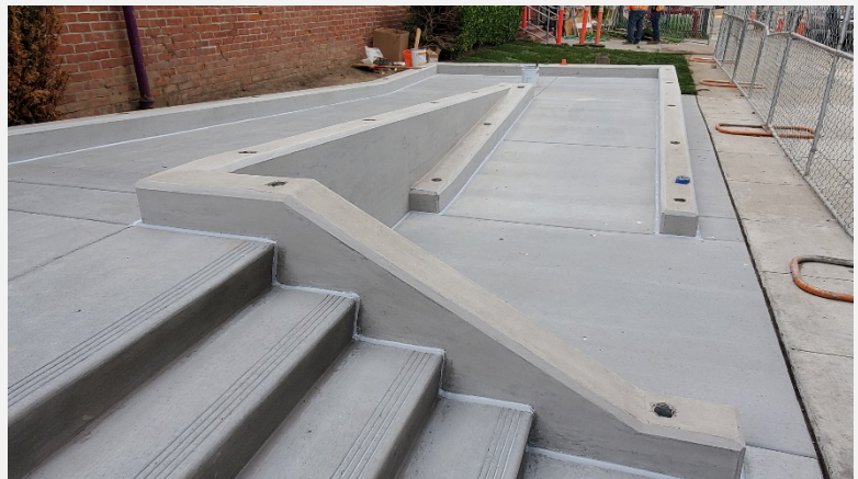
ADA accessible ramp installed at school entrance
