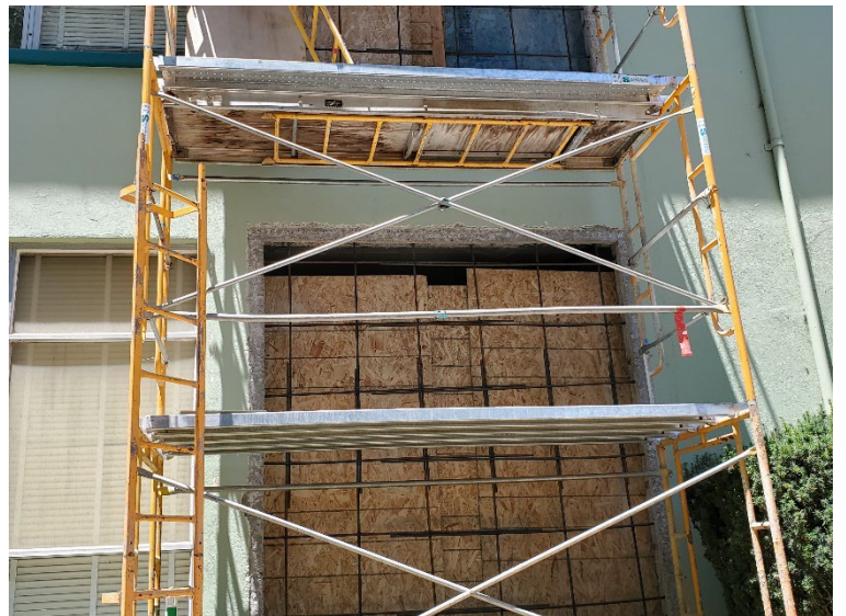
Glass block window – removal of existing caulking
