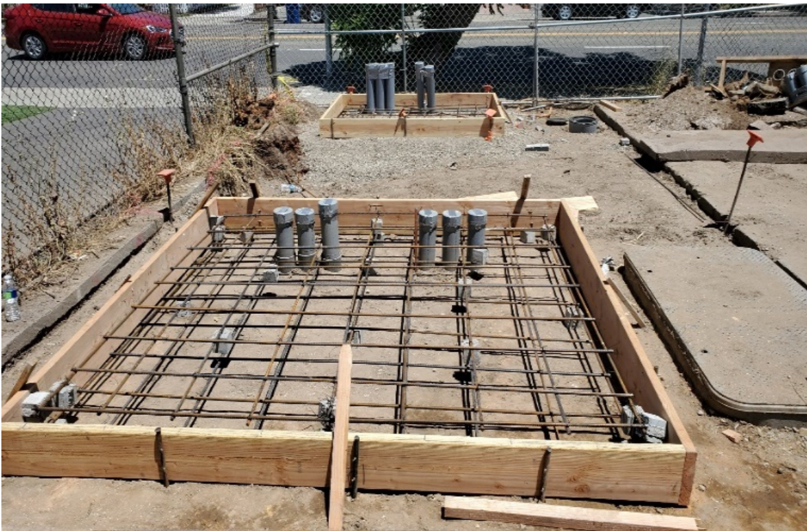
Preparation for new electrical service upgrade to entire school
