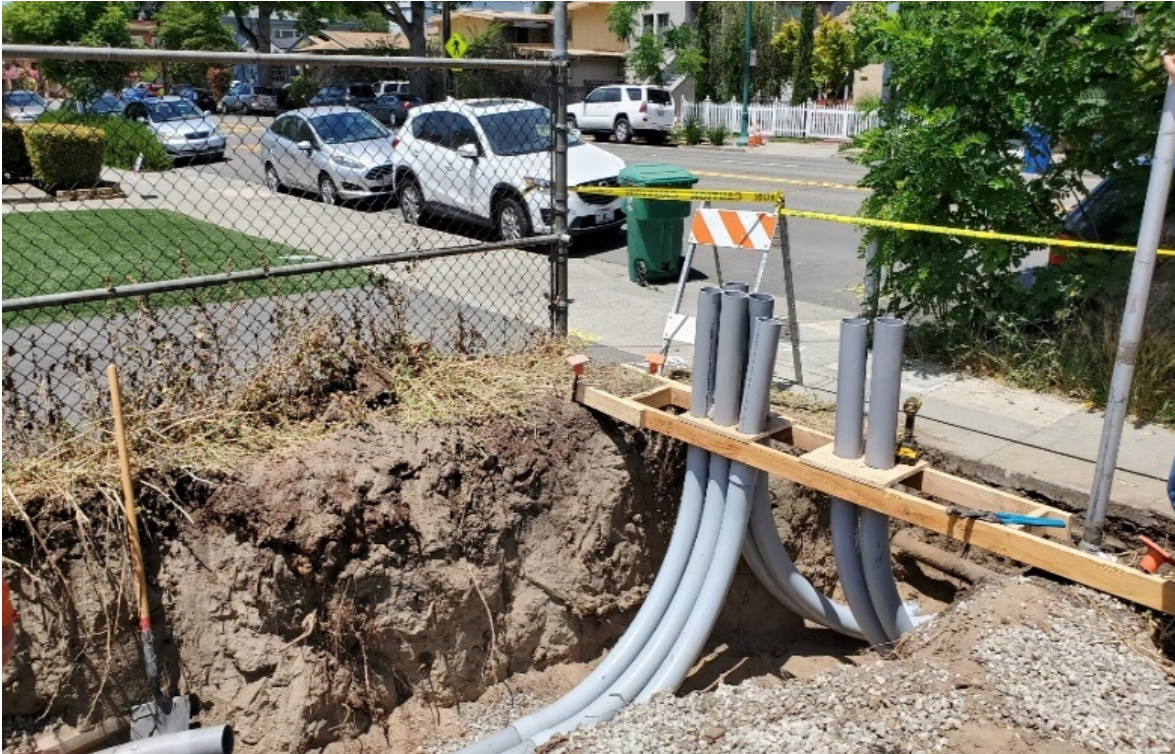
New Transformer – Conduit installation before concrete pad
