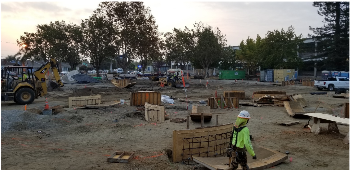
200 Building – Bench installation in progress at front quad
