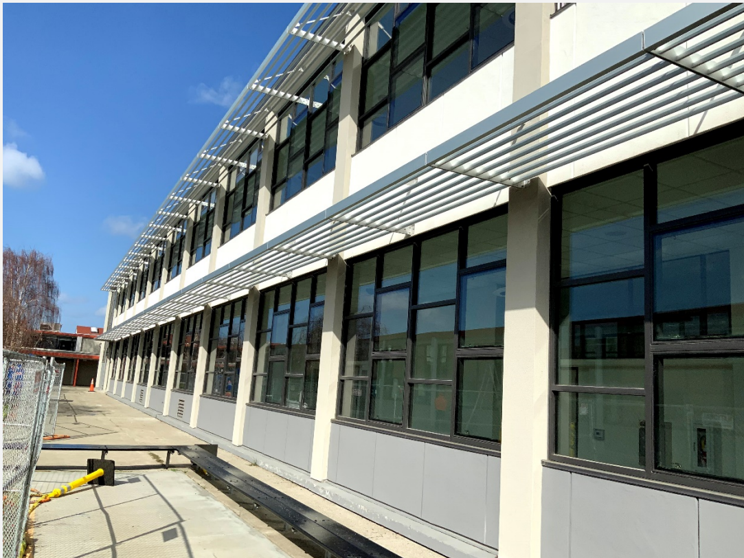
New windows and sunshades installed on Building 200
