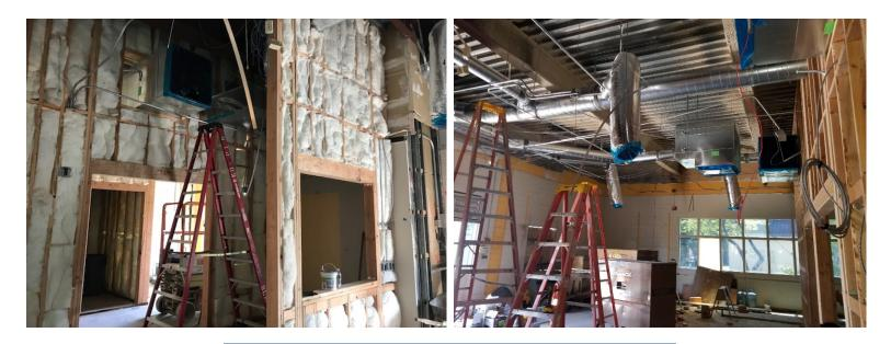
Admin Office framing, insulation & HVAC duct work
