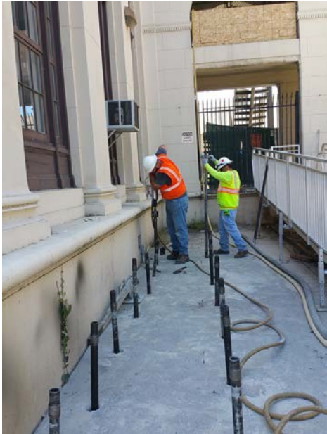
Grout injection, exterior & interior
