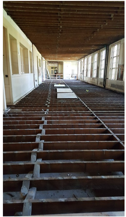
Post-abatement demolition in preparation for seismic mitigation
