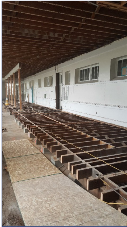
Post-abatement demolition in preparation for seismic mitigation
