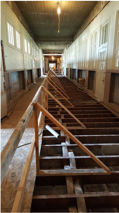
Post-abatement demolition in preparation for seismic mitigation
