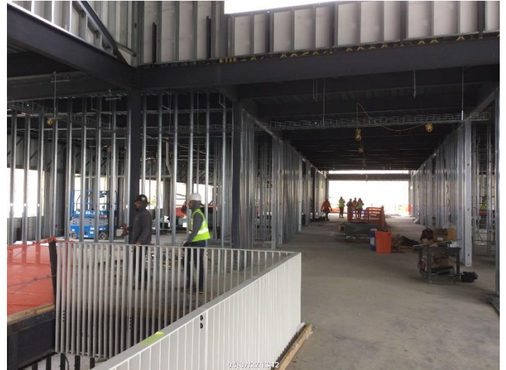
2 nd floor Interior Framing
