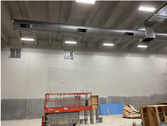
Gym painting and duct installation
