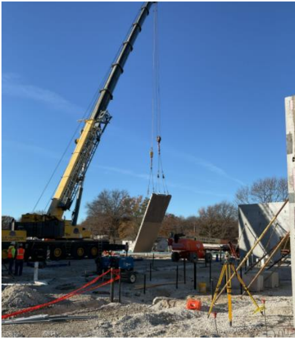
Picking Precast Panel
