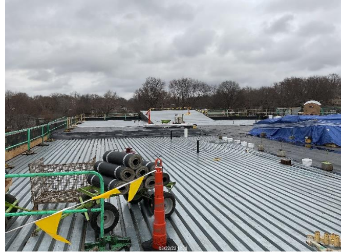
Area D Steel Roof Decking
