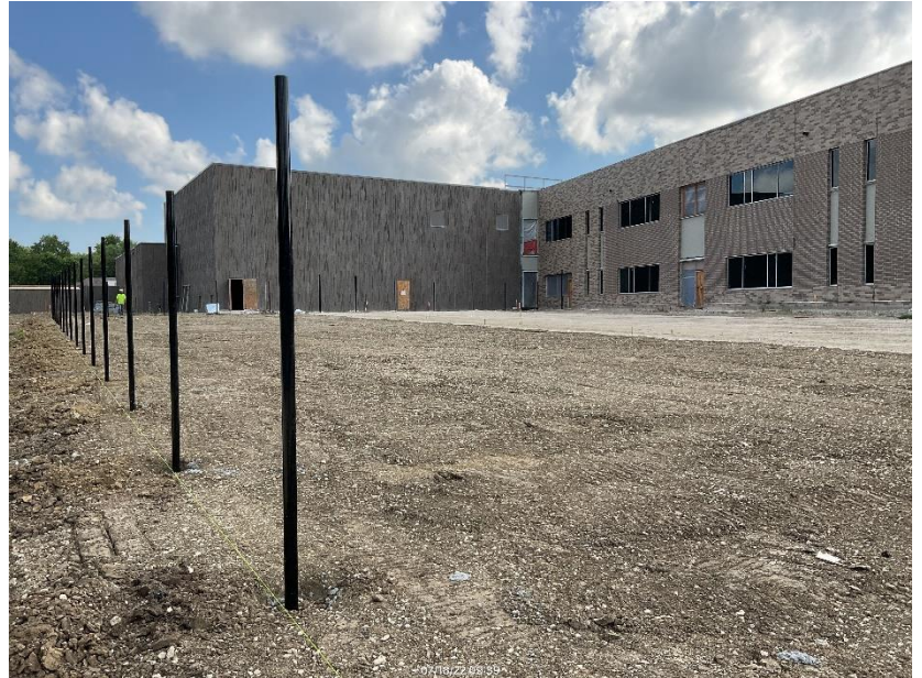
Grading and fence post installation of southwest side
