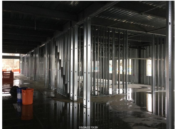
2 nd floor Interior Framing
