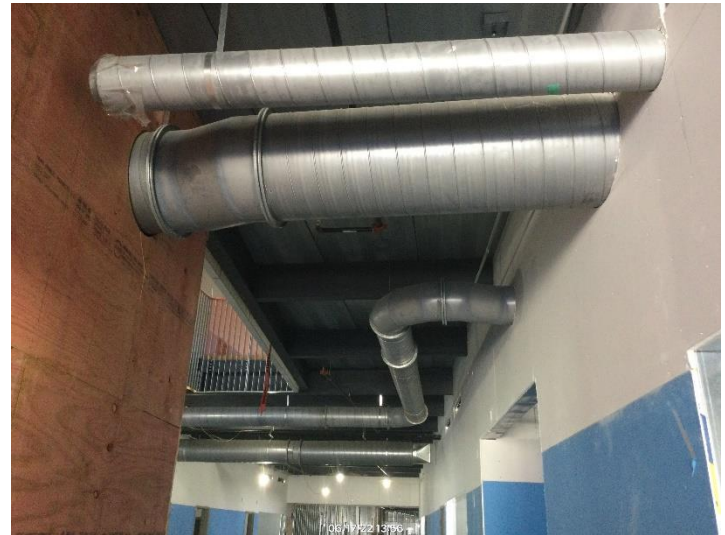
Ductwork Installation
