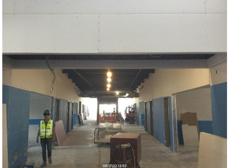
Area D Drywall installation
