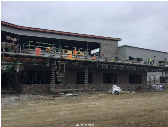
Area B brick masonry installation
