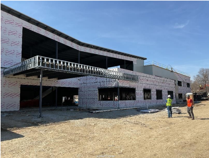
Area B sheathing and exterior spray air barrier installation
