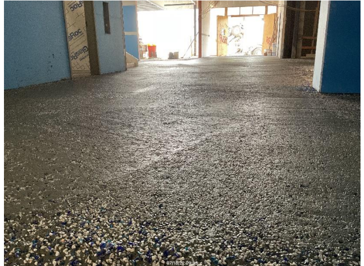
Laying of polished concrete topping slab in 1 st floor area B
