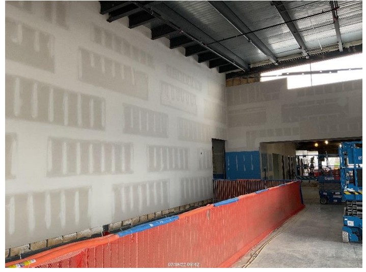
Area B drywall finishing
