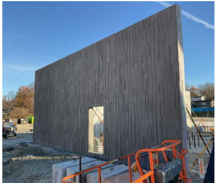
Exterior Precast Formliner
