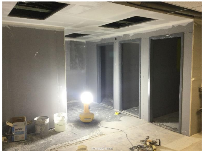
Continuing drywall installation in 2 nd floor bathrooms
