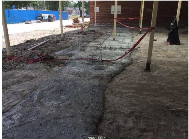
Poured footing in 2 nd floor addition
