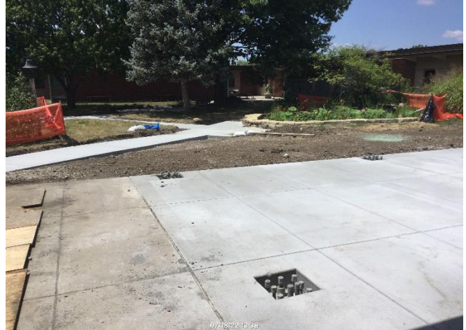
Poured new sidewalk and slab in courtyard area
