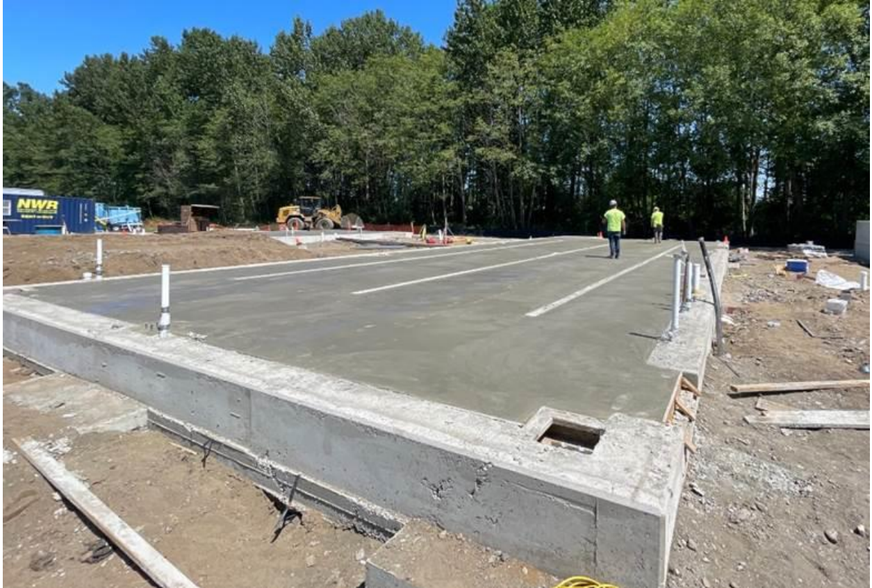
Floor slab poured at the Agriculture Science building
