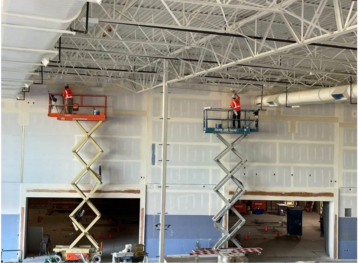
Final preparation of the sheetrock in the large commons gathering space
