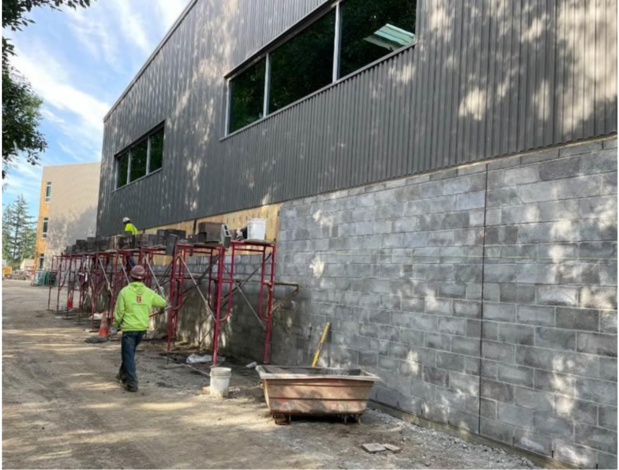
Masonry block around the back side of the Auxiliary Gym
