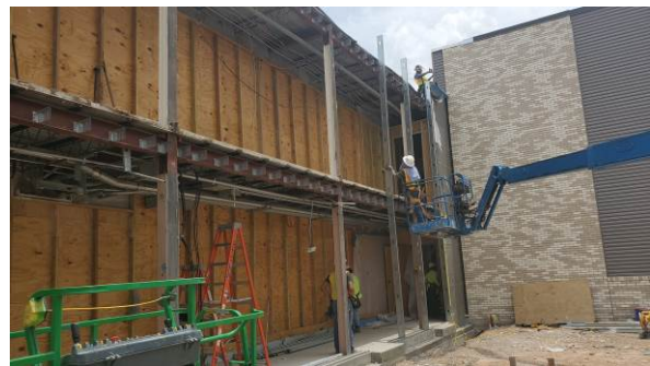
Area L exterior walls
