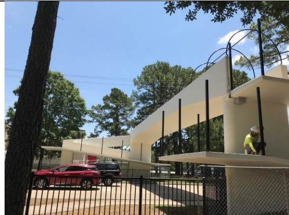
Existing bridge (new railings)
