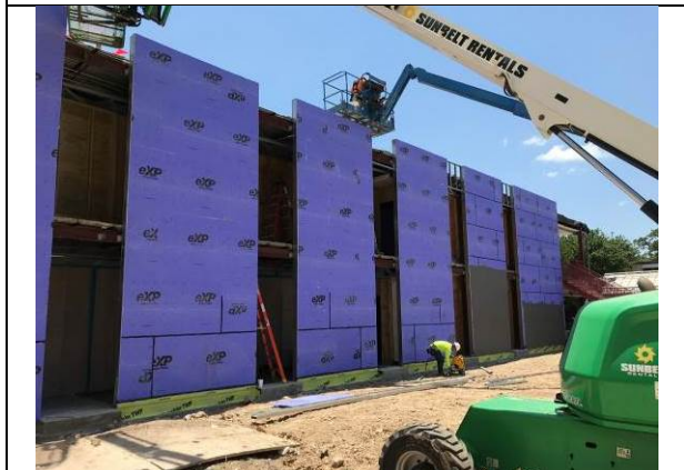
Area L exterior walls
