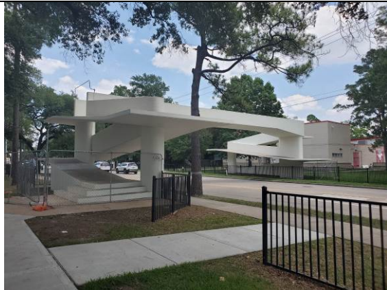
Existing bridge (repainted)
