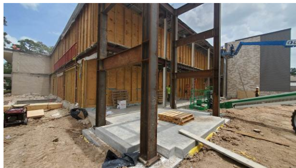
Area L framing for new entry
