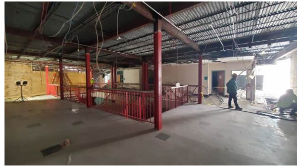
Area L interior renovations
