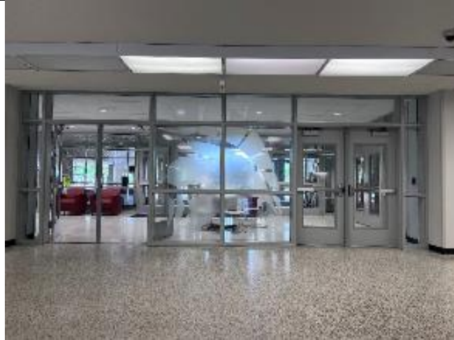
Overall view of Main Entry from Dining.
