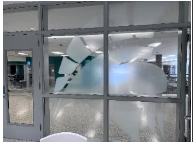
Logo film has been applied to glazing at existing lobby.
