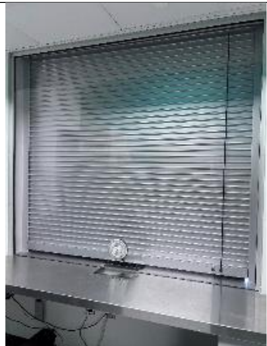
Ticket Booth glazing has been installed.
