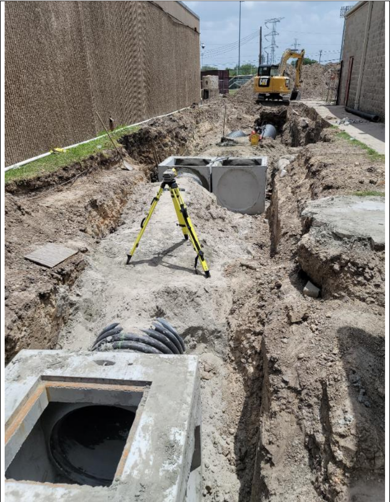
Athletic alley scope of work is ongoing.
