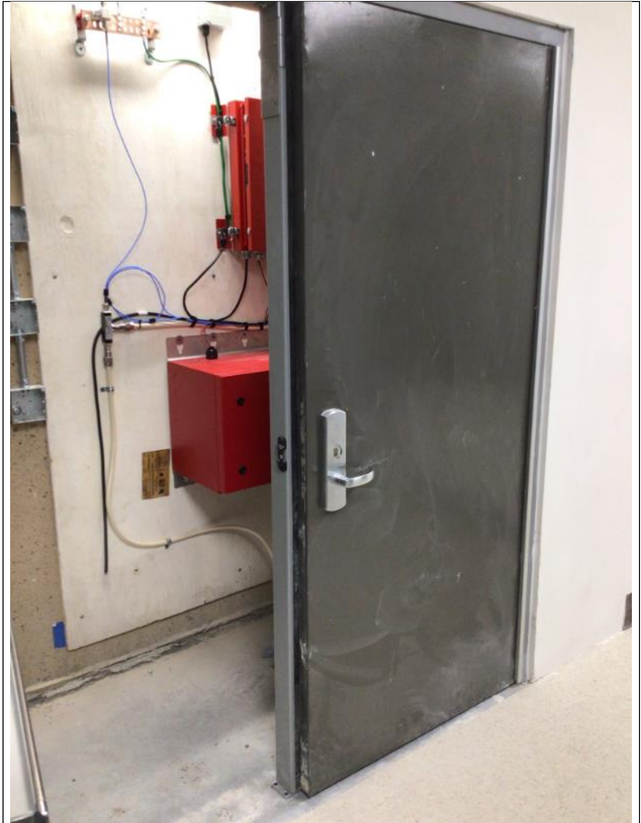
ERRC scope of work is nearing completion.
