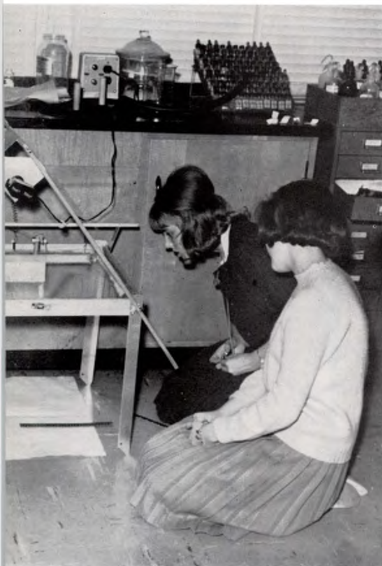
Measuring wave lengths, Ruth Bardolph and Mary Stob work on a ripple tank experiment.
