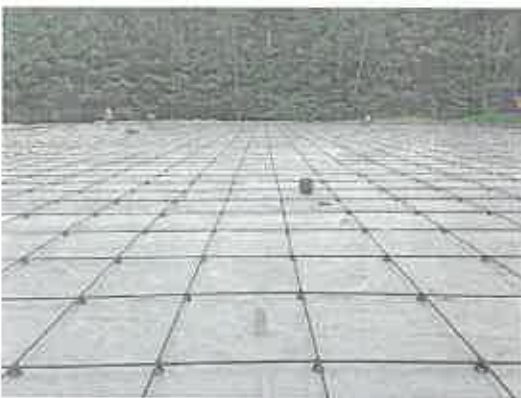
Cable Layout Prior to Concrete Installation
