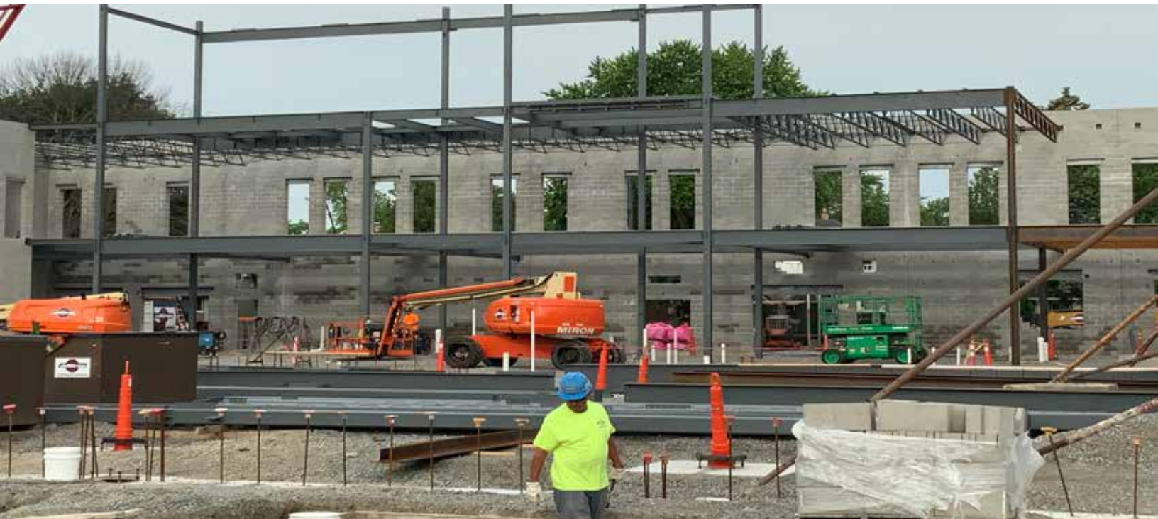
STEEL RISING WITHIN THE WEST PORTION OF VEL PHILLIPS MIDDLE SCHOOL
