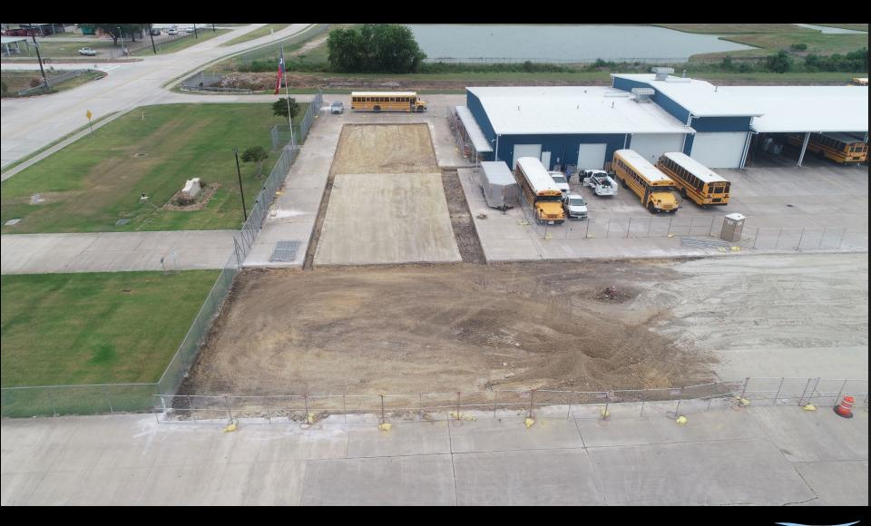
cre 8 Concrete Saw Cut & Sub Grade Prep In Progress for New Fuel Station
