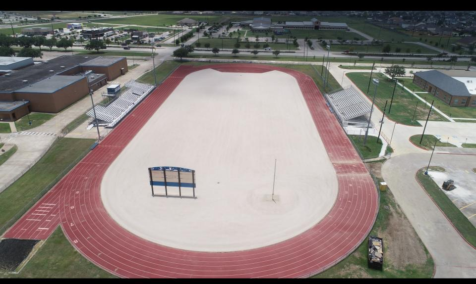
Artificial Turf – Track Resurface – Subgrade, Liner & Gravel Complete – Artificial Turf Installation to Begin by 6-28-22
