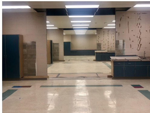
Classroom openings will allow for an increase in collaboration and flexibility for both small group and large group learning. Three classrooms are shown with their new connections created.
