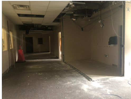
Demolition in the planned reception and office area
