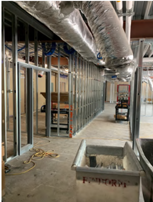
Steel Stud Framed Walls of Office Spaces
