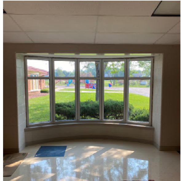
Newly Installed Aluminum Framed Windows
