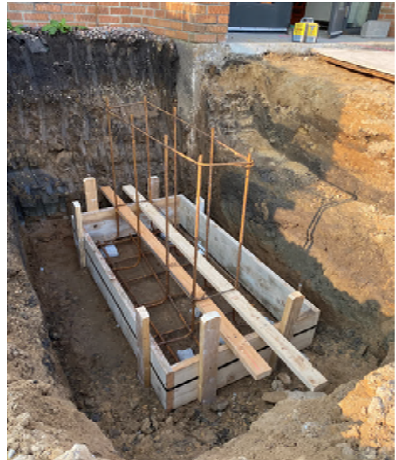
Concrete Formwork for New Entry Columns
