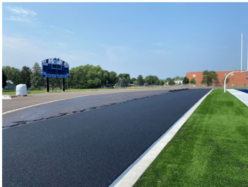
First Layer of Track Surface
