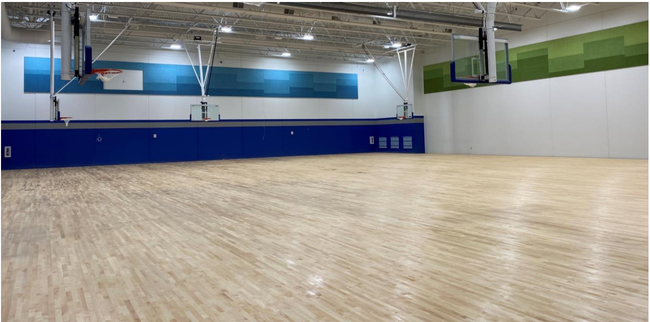
Gym Floor After First Coat of Finish
