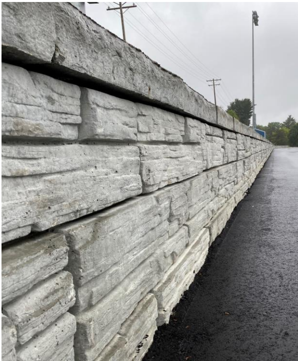
Visitor Side Block Retaining Wall
