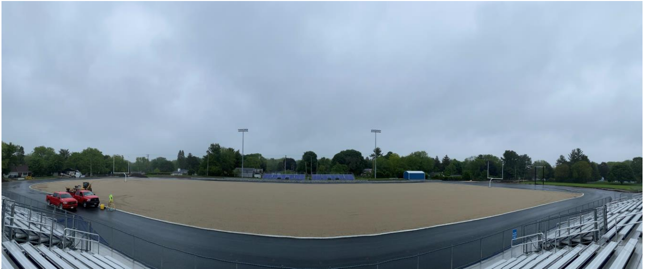
Binder Course of Track
