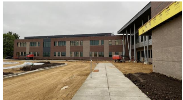
Front Entrance Sidewalk
