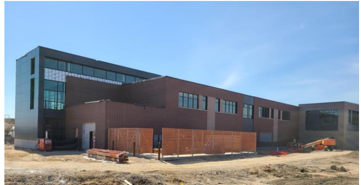
Area B/Trash Enclosure
