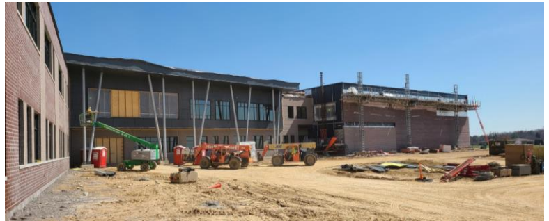
Area C Main Entrance
