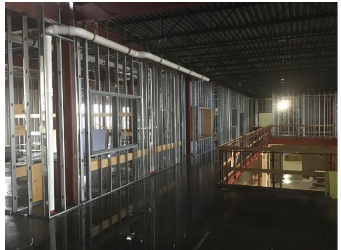
Level 2 Area C interior walls have been framed.
