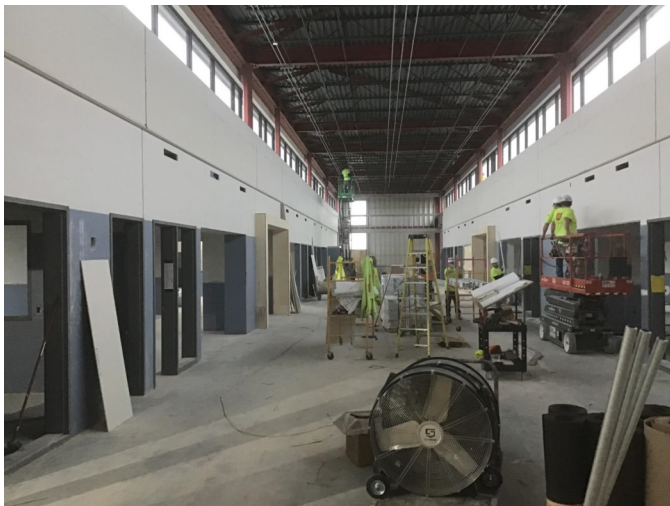
Level 2 Area B drywall installation.
