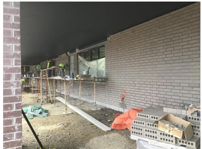
Brick Installation on Bus drop off entryway (South side of Area B).
