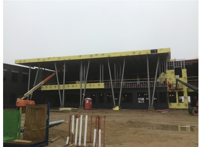
Entryway Canopy studs and sheathing.
