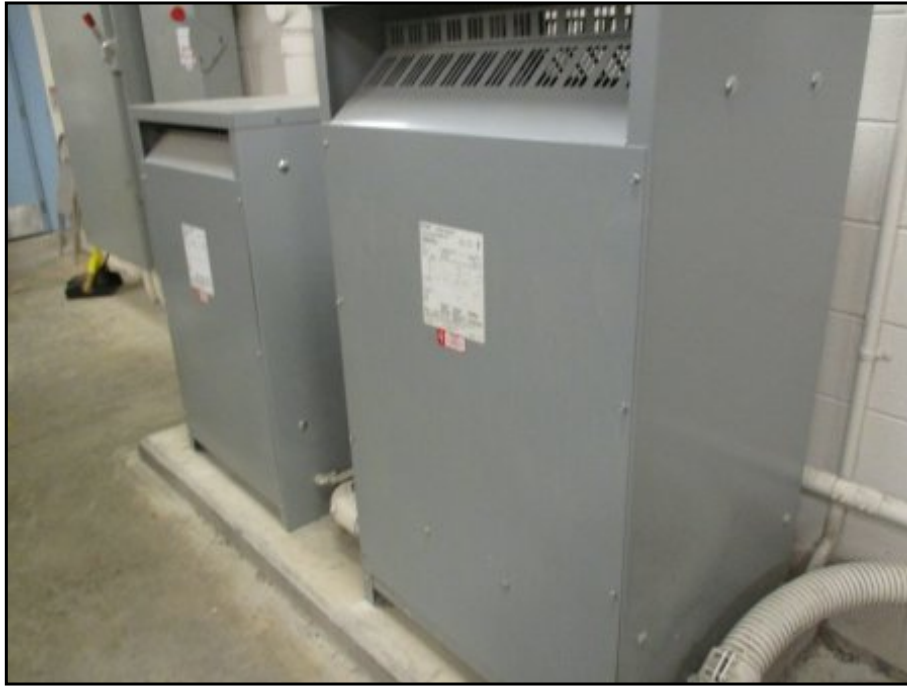
View of the two pad-mounted transformers located in the mechanical room of the main building on the Property.
