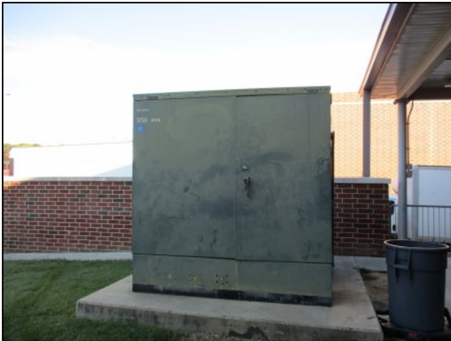
View of the main pad-mounted transformer for the building located on the southwestern exterior of the main building on the Property.
