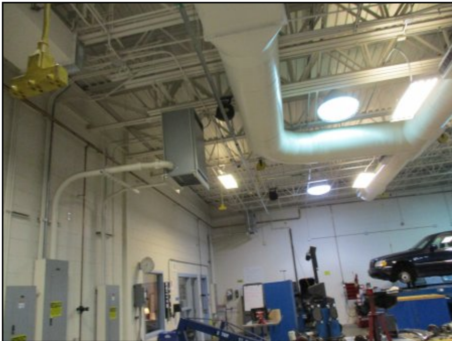
View of the electric heaters to the autoshop in the main building on the Property.
