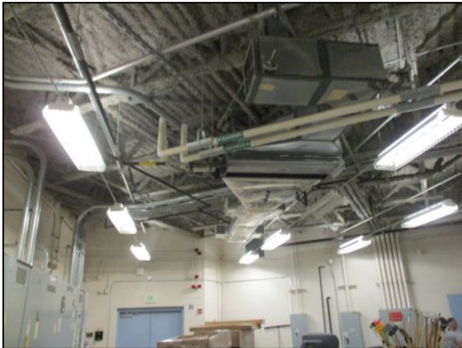
View of the electric heating units for the maintenance room of the main building on the Property.
