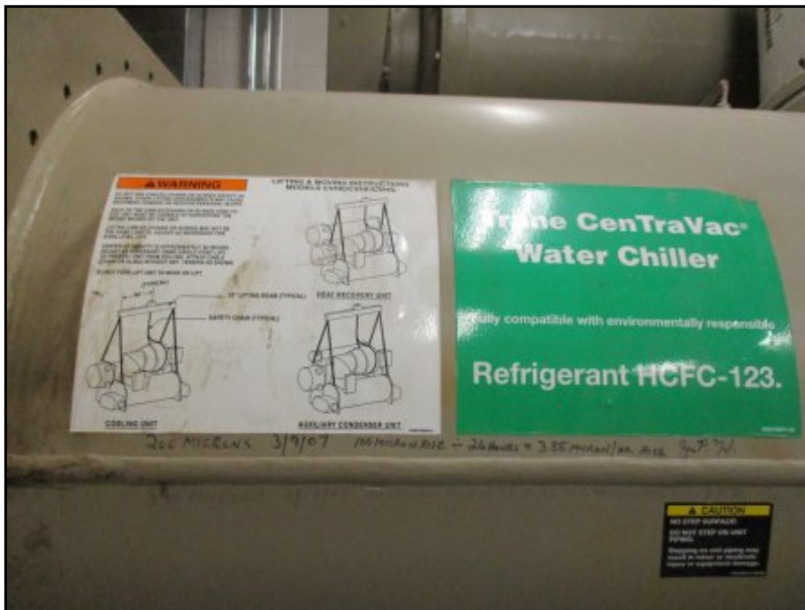
View of the main water chiller in the boiler room of the main building on the Property.
